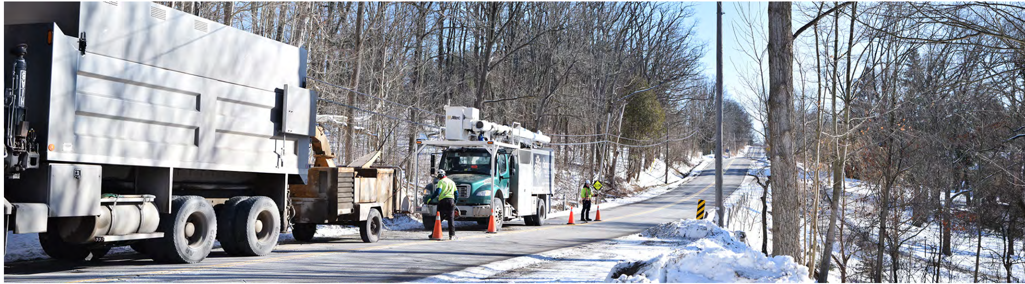
Photo 42: 5390 Cedar Springs Road. Facing Towards Proposed Western Extension.
