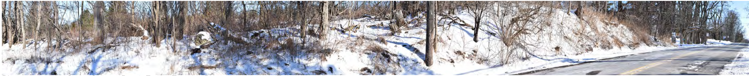
Photo 35: 5264 Cedar Springs Road. Facing Towards Proposed Western Extension.
