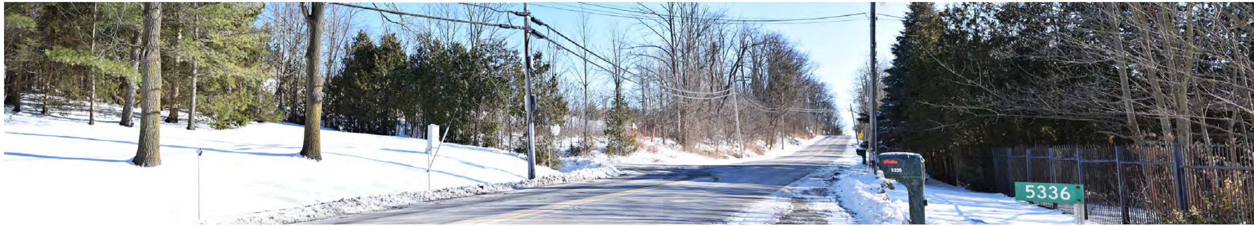
Photo 39: 5336 Cedar Springs Road. Facing Towards Proposed Western Extension.
