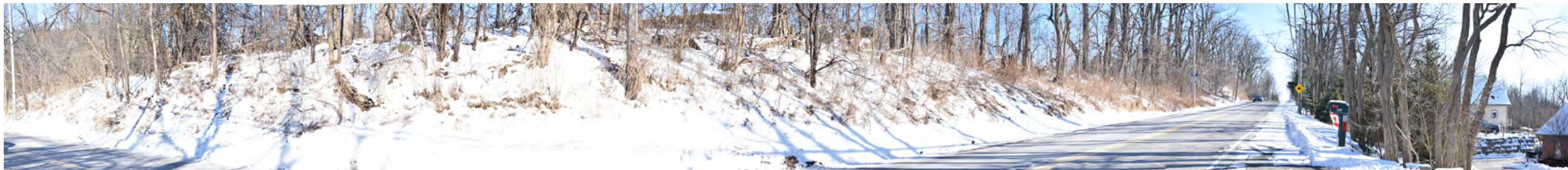
Photo 36: 5268 Cedar Springs Road. Facing Towards Proposed Western Extension.
