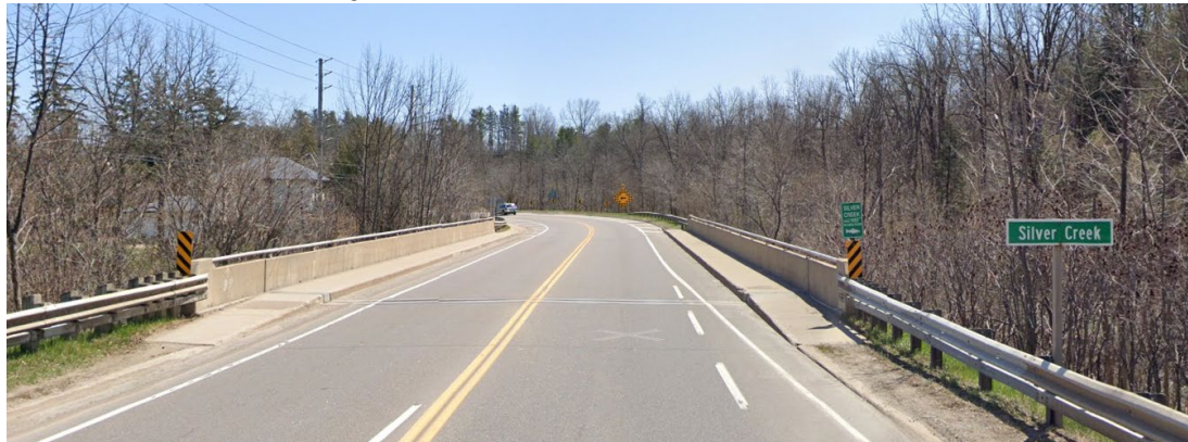
Silver Creek Structure (July 2022)
