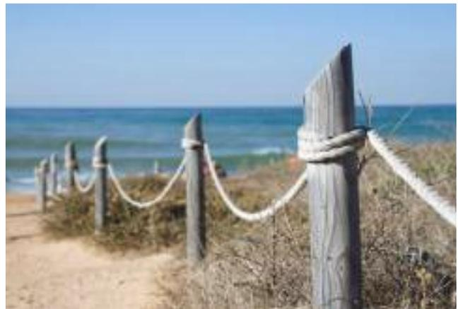
**Figure 5.0.1** - Example of post and rope to protect beach dunes.
