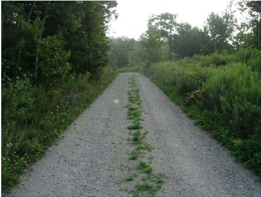
Photo 3 – A view of the East Cell watermain and driving access. In areas where the alignment crossed through old field areas, the shoulder and safety berm (on the right side of the access in this photo) were seeded with a standard MTO seed mix. The extraction area is off to the right.
