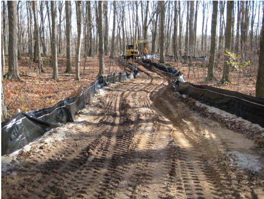
Photo 13 – View showing the buried feeder line to Recharge Well RW317D, after backfilling. Extra feeder lines are typically buried at the same time; if additional recharge wells are subsequently required then less trenching will be necessary. GHD 2012-11-14
