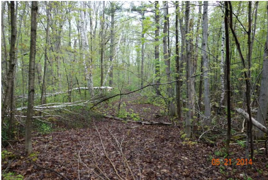
Photo 19 – View of the feeder line leading to Recharge Well RW201B, taken 5 years after the feeder line was buried in 2009. GHD 2014-05-21
