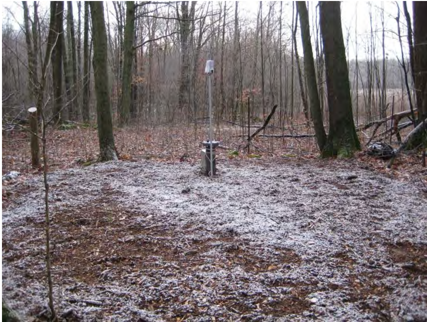
Photo 29 – View showing Recharge Well RW316C shortly after installation in late 2012. Note the 15-20 cm deep layer of fresh wood chips that were placed on the disturbed area.
