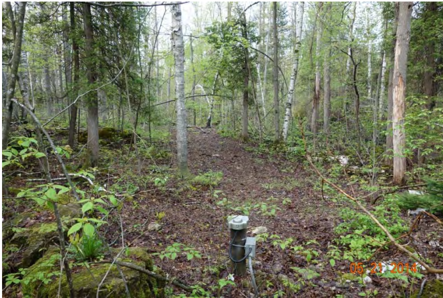
Photo 33 – View of Recharge Well RW207C, taken 5 years after installation in 2009. Note the regeneration of Alternate-leaved Dogwood, Bracken and sedges. GHD 2014-05-21
