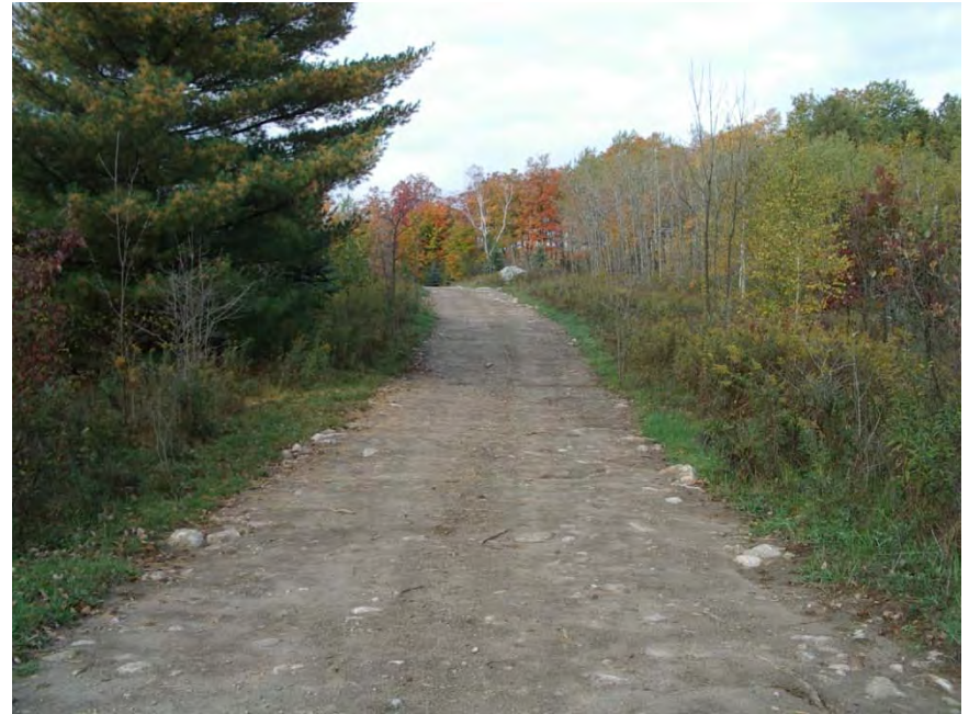
Photo 8 – Second view showing recently buried feeder lines leading to Recharge Wells RW203C, RW203D, RW204C and RW204D, closer to Sixth Line. GEC 2012-10-09
