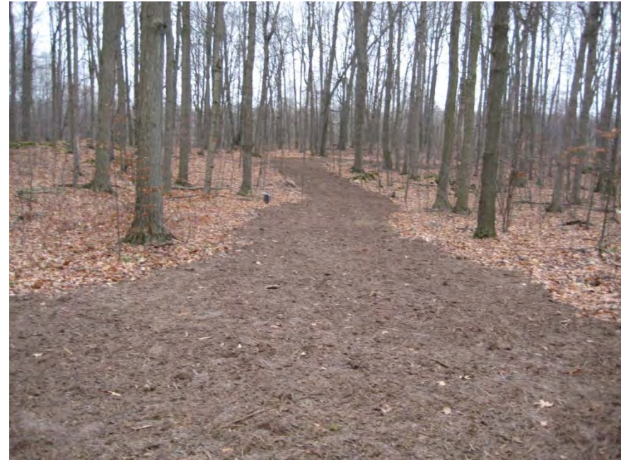
Photo 14 – This is the same view of buried feeder lines to Recharge Well RW317D, after restoration. The 15 to 20 cm deep layer of wood chips helps to prevent the establishment and spread of invasive groundcover species such as Garlic Mustard ( Alliaria petiolata ). GHD 2012-11-30
