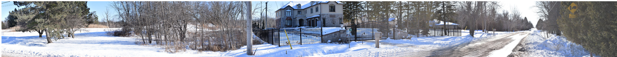
Photo 49: 2473 2 Side Road. Facing Towards Proposed Southern Extension.
