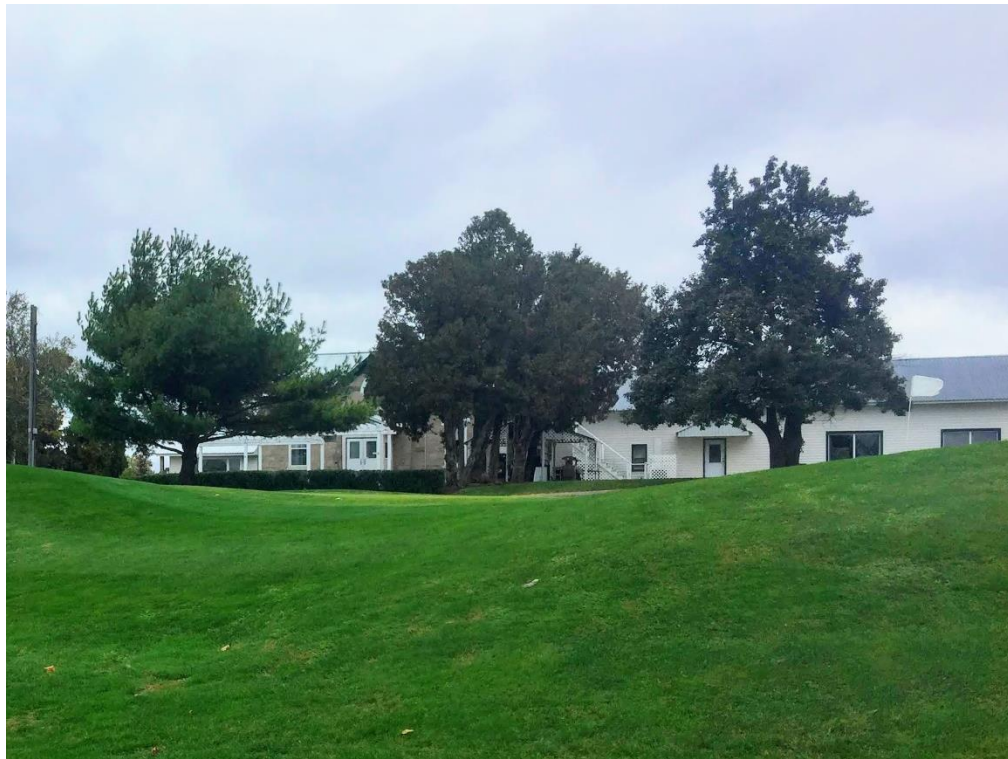
Image 1 Looking northeast at disturbances associated with the existing Burlington Springs Golf Club clubhouse.
