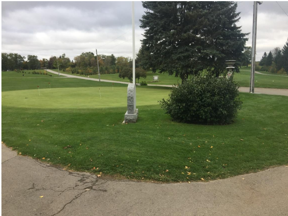
Image 5 Looking southwest at disturbances associated with USGA putting greens, paved access road and pathway.
