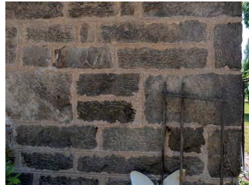
Figure 18: Typical masonry tooling, coursing and pointing as seen on the north elevation.
