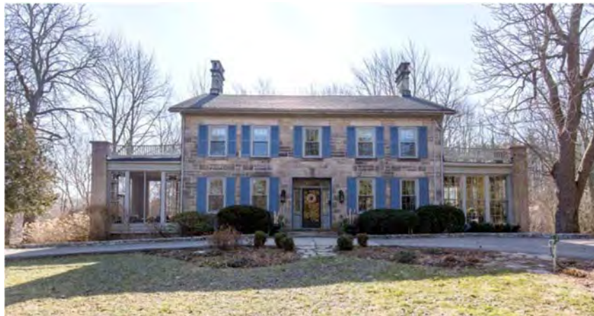
Figure 31: The central portion of Springdale (b.1810) outside Dundas, Ontario demonstrates the massing, form and composition typical of the Georgian style in Ontario. Incidentally the house employs a similar coursing to that of the subject property (Hamilton Built Heritage Inventory Form for 6 Webster's Falls Road, Flamborough).
