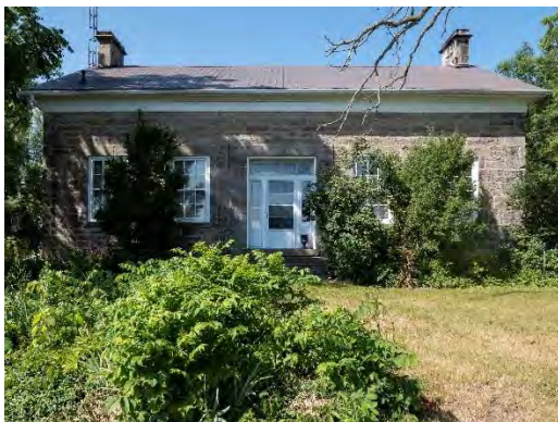
Figure 11: The east elevation of the farmhouse displays a formal symmetry accentuated by its restrained decorative regimen.
