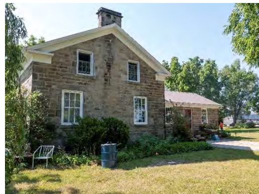
Figure 12: The north elevation is again defined by symmetry and proportion. The entrance off the rear wing is formal in design despite its secondary nature.
