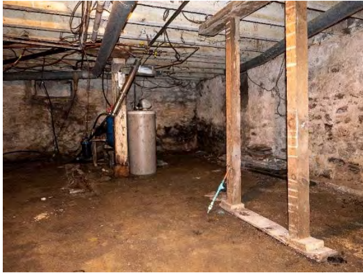
Figure 23: View northwest of the basement under the rear wing, with evidence of former plaster walls visible on remaining posts.
