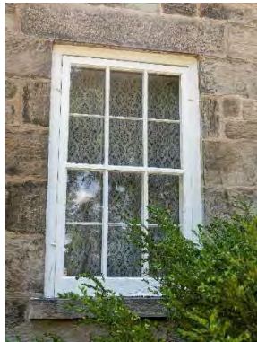
Figure 17: Typical historic window configuration on the north elevation, with six-over-six double hung sash covered by a storm window.
