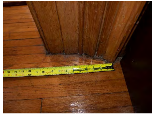
Figure 26: The profile of the typical Grecian ogee is seen in the living room, roughly between the 1 1/4" and 4 3/4" marks on the tape measure.
