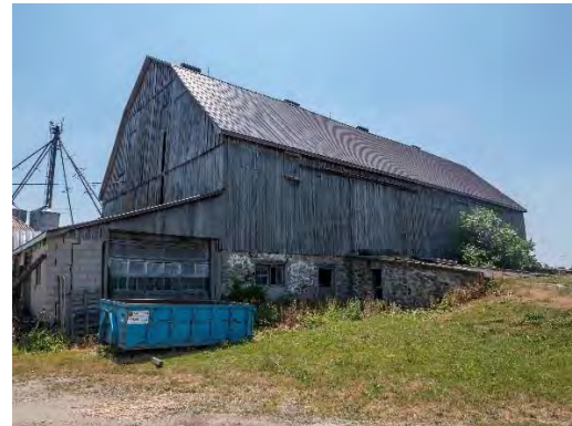
Figure 8: Looking southwest at the two-storey barn, showing raised embankment to the second storey entrance and shed roof addition at the left.
