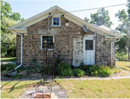
Figure 15: The rear wall of the rear wing has a slightly modified roof profile and whitewash from a former addition.
