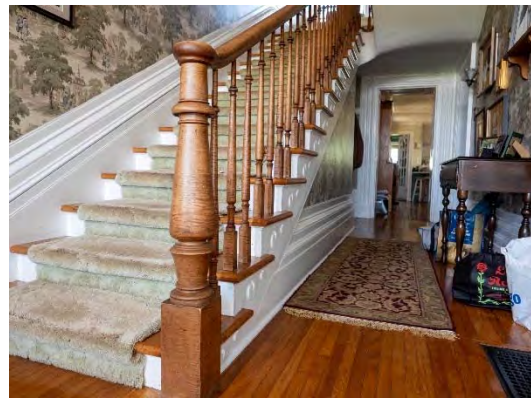
Figure 20: The staircase dominates the central hall with its prominent curly maple figuring.
