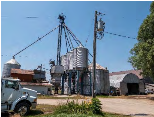
Figure 7: The grain silo complex includes hoppers and silos connected via conveyor system, and a scale house all clad in metal.
