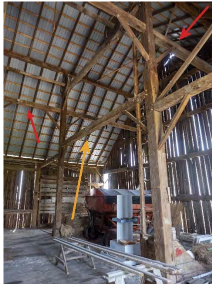
Figure 10: The three-bay bent design of the barn is similar to that of Radford's Dairy Bank Barn, with notable differences in the proportion of bays, the use of an offset beam (orange arrow), and an additional girder below the upper top sills (red arrows).
