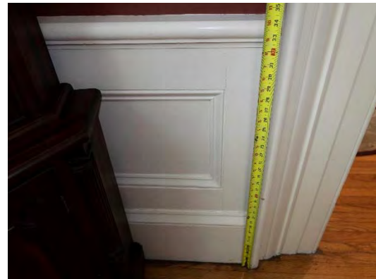
Figure 28: Typical wainscoting in the dining room is an embellishing version of that in the kitchen.
