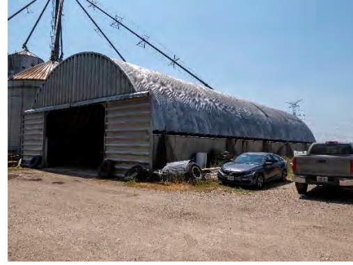
Figure 6: The quonset hut storage structure sits between the barn (to the right) and grain silo complex to the left.
