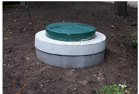
Photo courtesy of Simon Smith Drilling Ltd.
