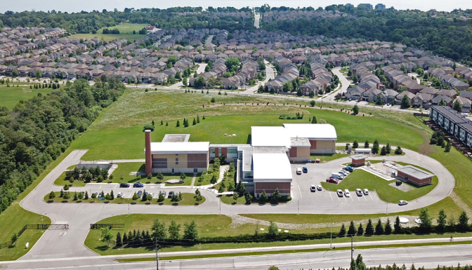
Burloak Water Treatment Plant
