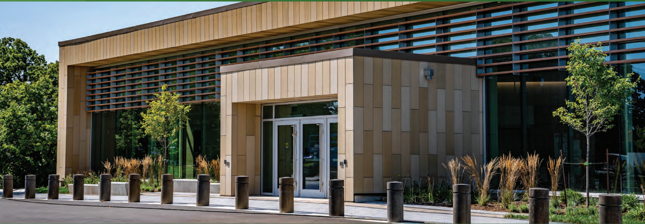
VIEW OF THE WEST ENTRANCE TO HALTON REGIONAL CENTRE
