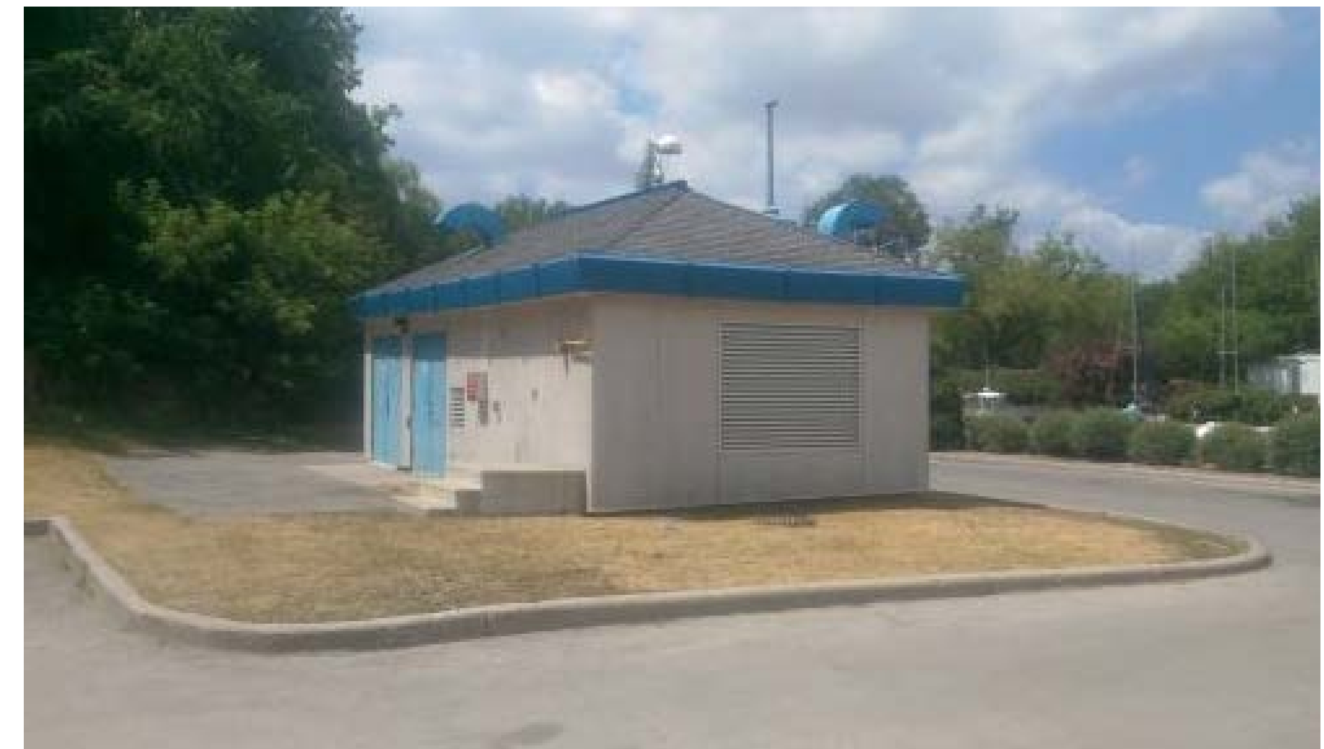
Pumping Station Building
