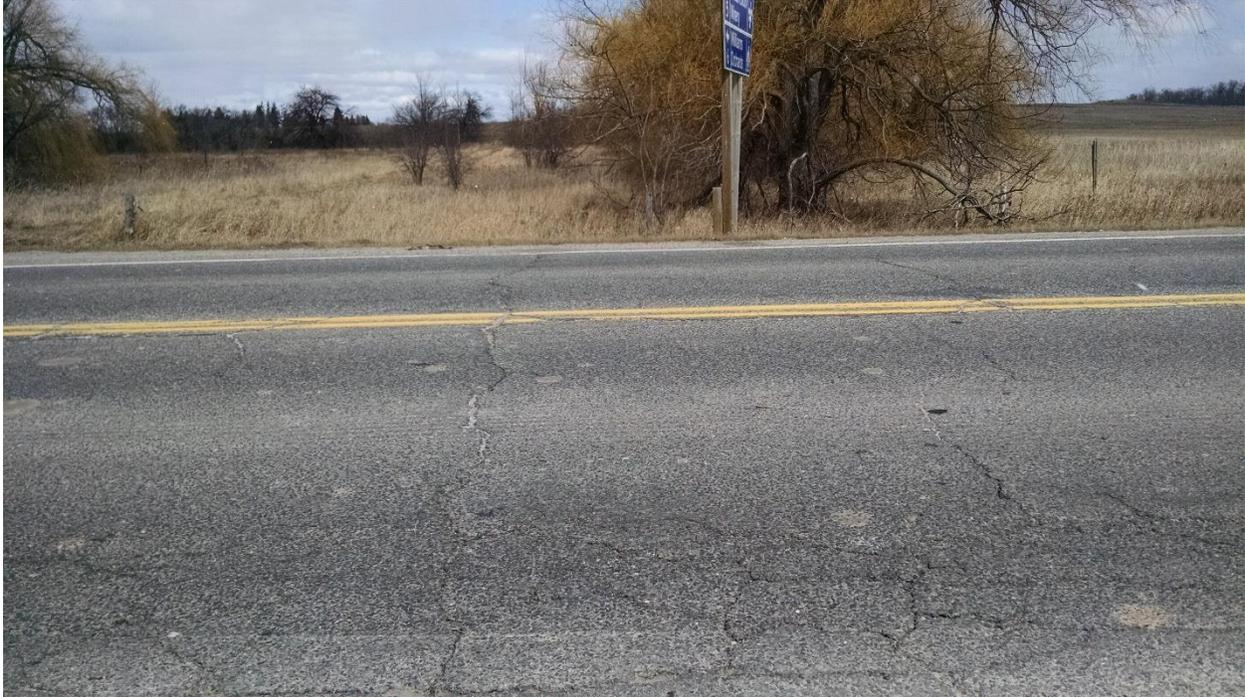
**Photograph 7 – Deteriorated Pavement Condition South of 10 Side Road**
