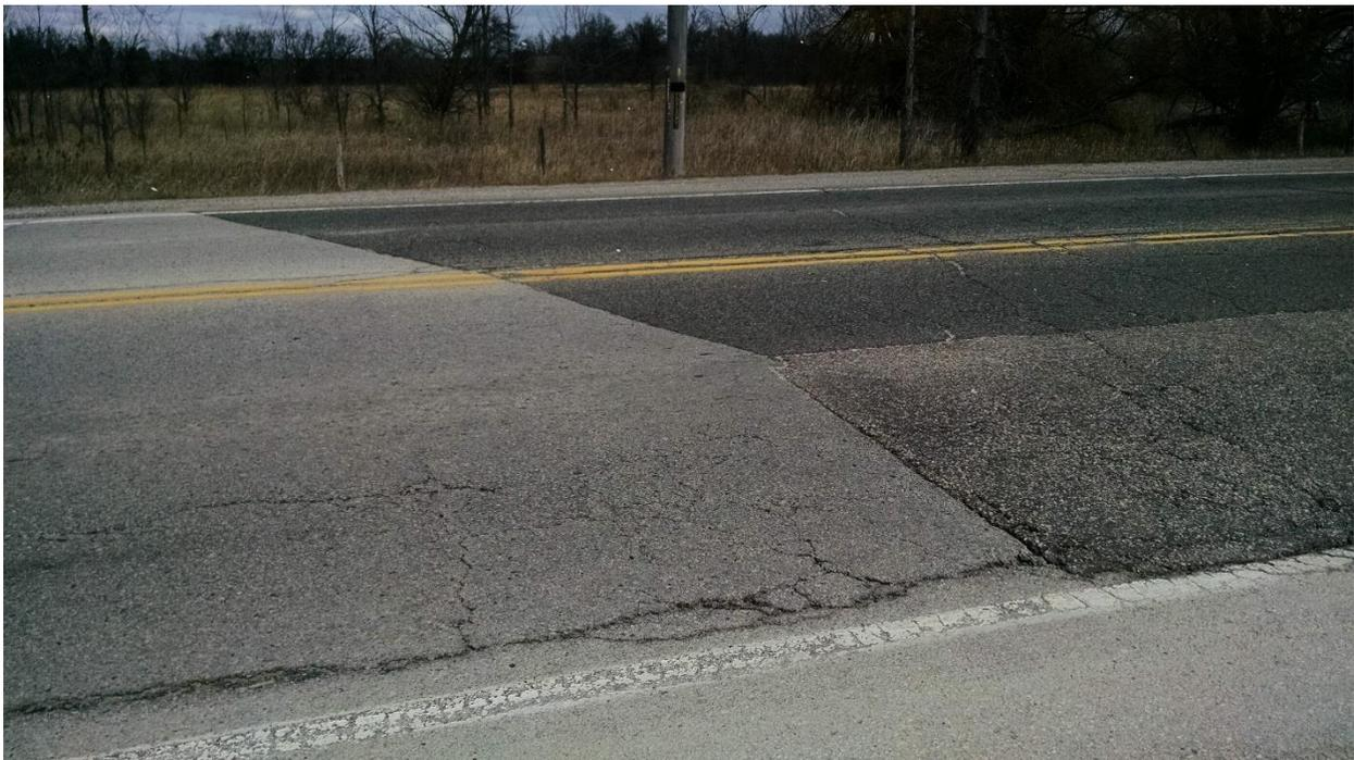
**Photograph 8 – Deteriorated Pavement Condition North of 10 Side Road**
