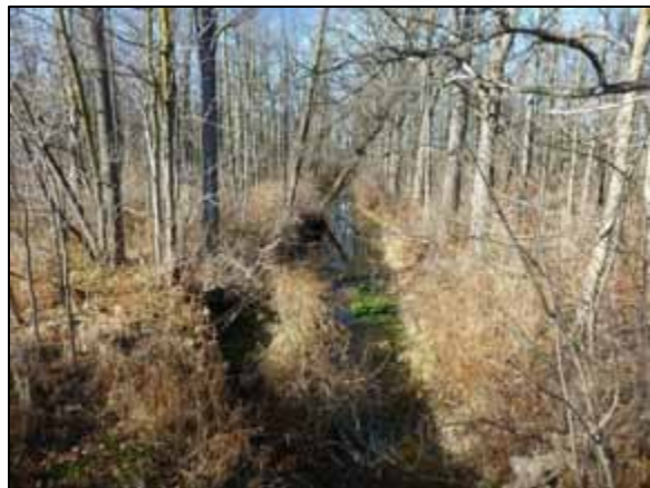
View upstream from inlet
