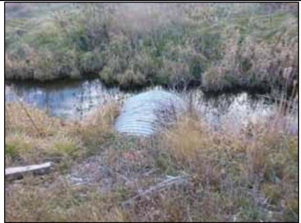
View upstream: culvert inlet
