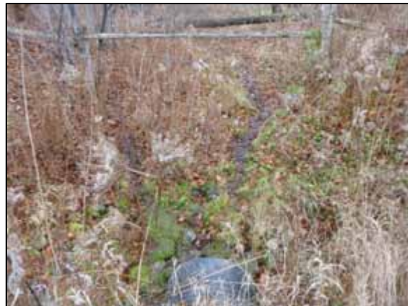
View upstream from inlet
