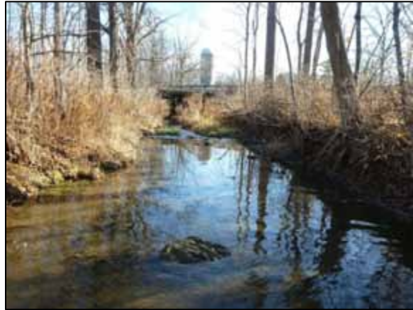
View looking downstream to C1 inlet
