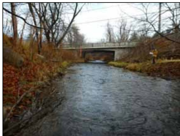
View downstream to inlet of Trafalgar Road bridge
