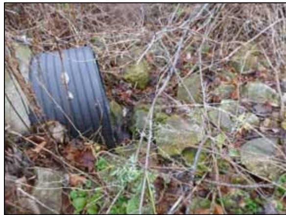
Outlet with bed protection
