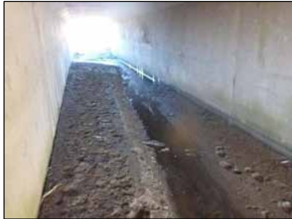
View inside of culvert
