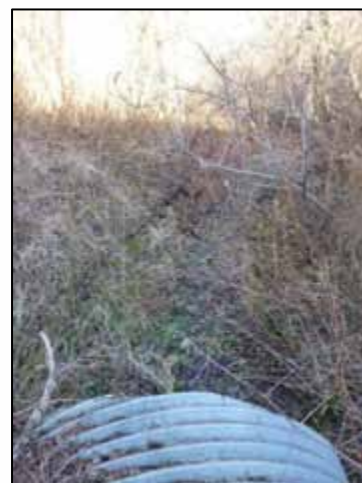
View downstream from culvert outlet
