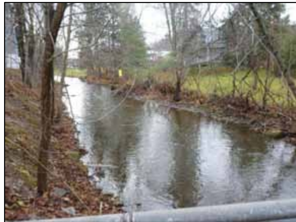
View upstream from Stewarttown Bridge
