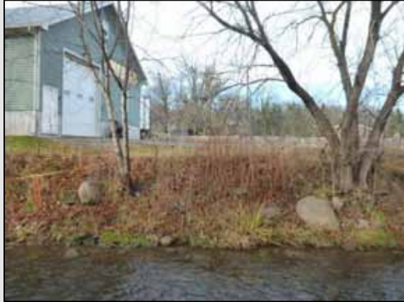
Left bank with large stone bank protection upstream of Trafalgar Road
