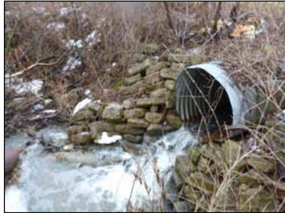
Outlet of access road culvert
