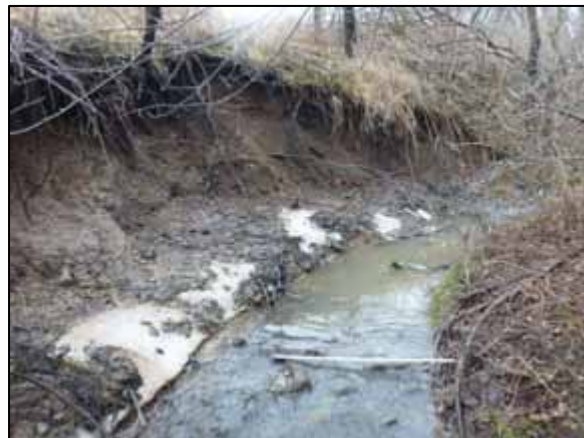
Erosion on western valley slope
