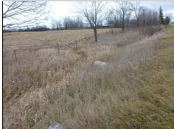
Ditch and agricultural swale looking upstream
