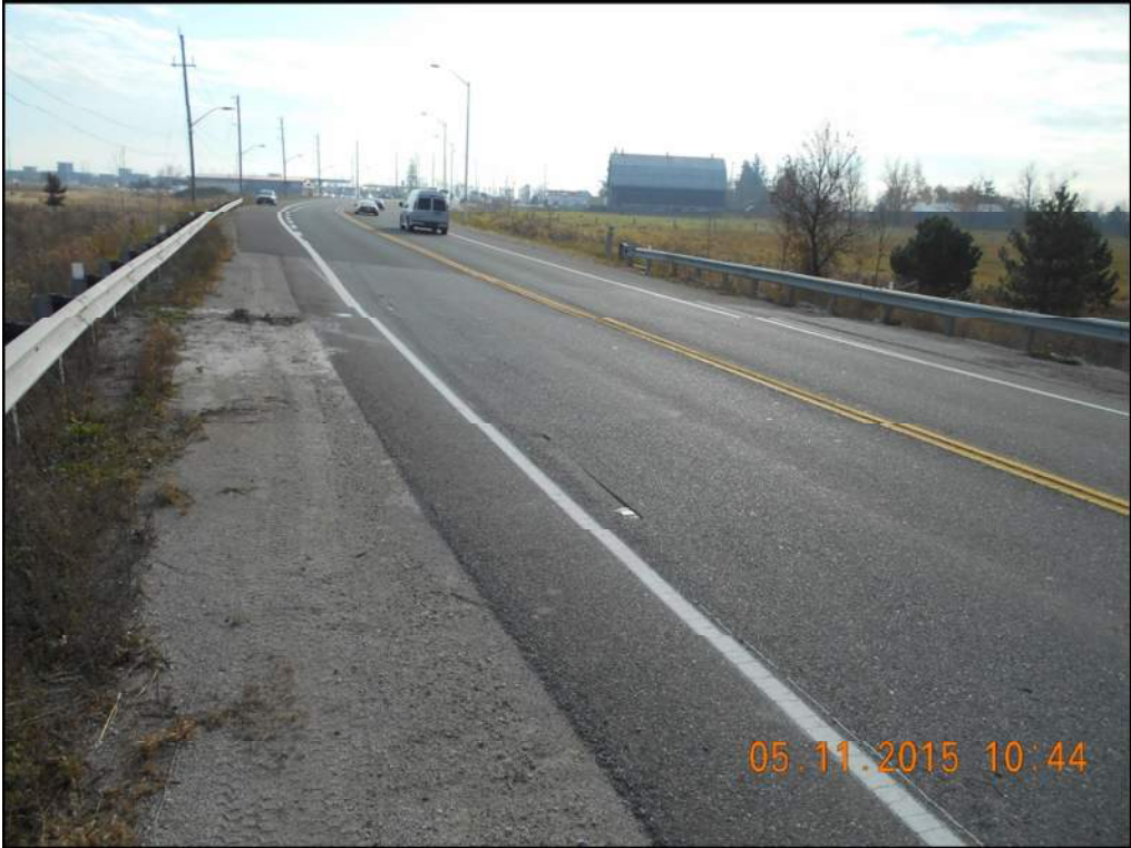
Photo 6: Approach Roadway above Culvert
