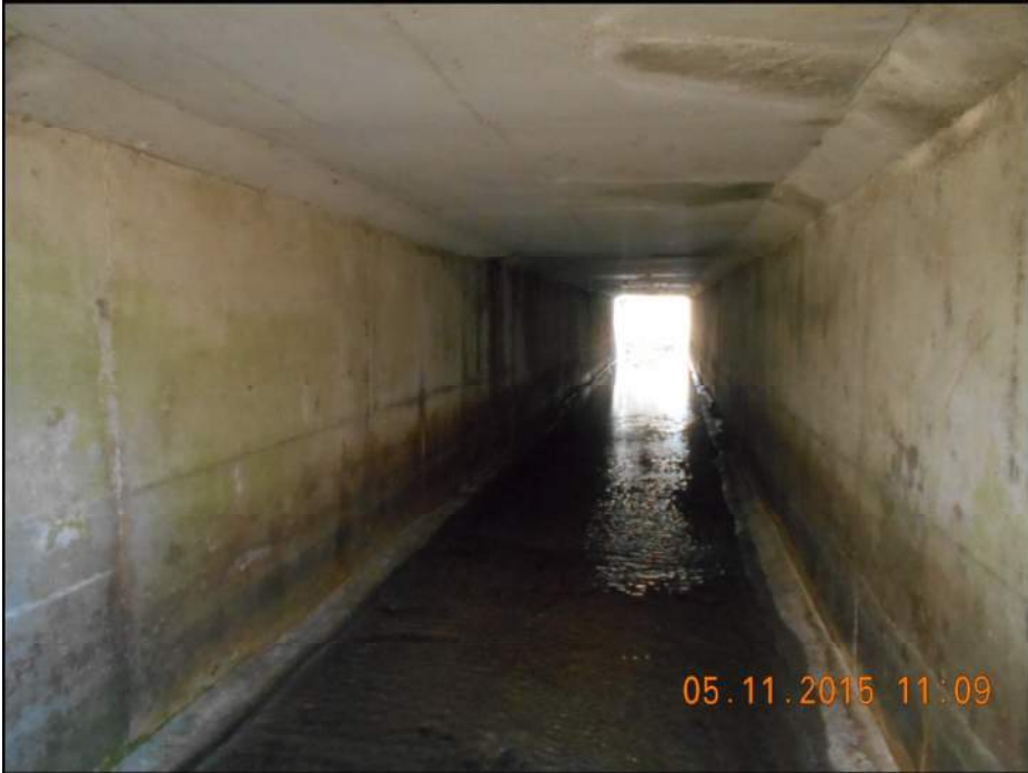
Photo 17: South Box Watercourse
