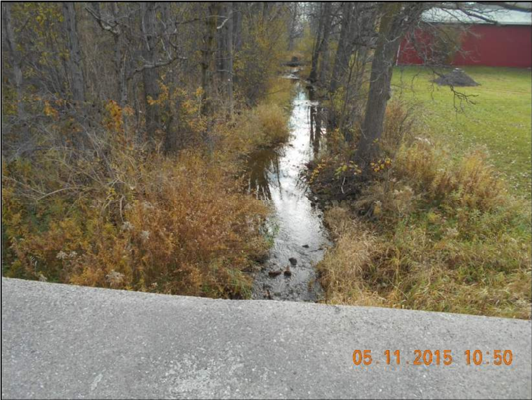
Photo 20: Downstream of Culvert
