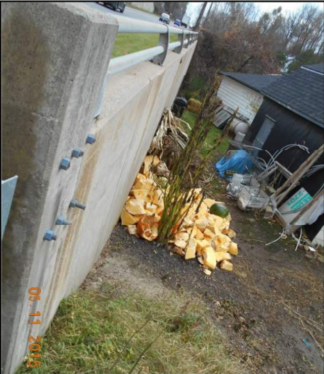
Photo 6: Retaining wall to the southwest
