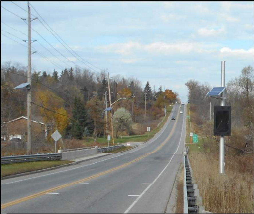
Photo 8: Looking north over structure
