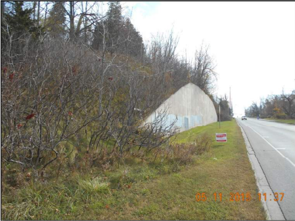
Photo 7: Retaining wall to the southeast
