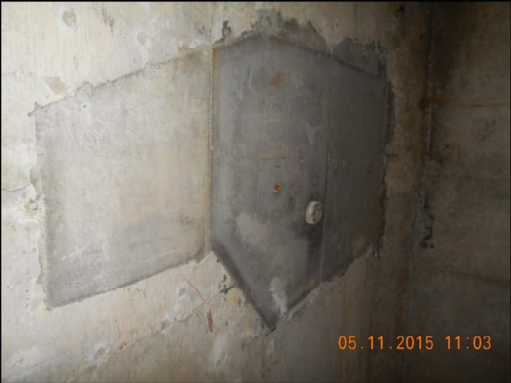
Photo 10: Soffit patch repairs (typical)
