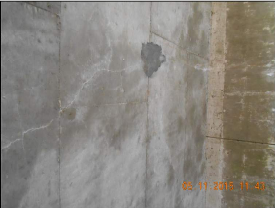
Photo 5: Soffit local patch repairs
