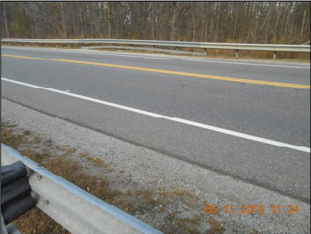
Photo 16: Asphalt Wearing Surface above Culvert
