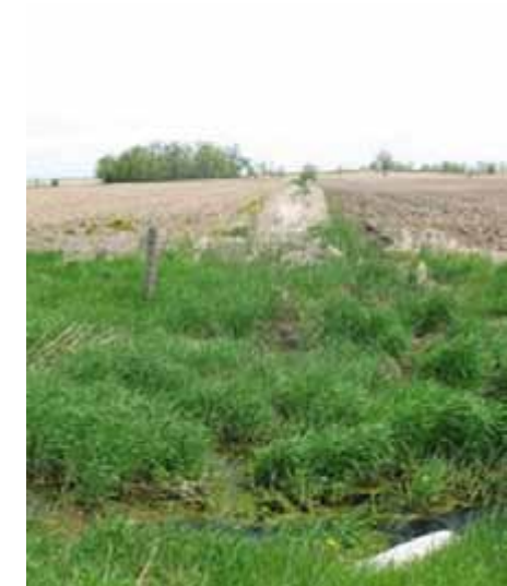
Feature 8: Watercourse Crossing – channelized drain. May 23, 2014.
