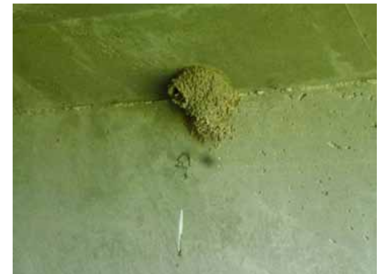
Feature 1: Cliff Swallow Nest on Culvert Structure. June 6, 2014.
