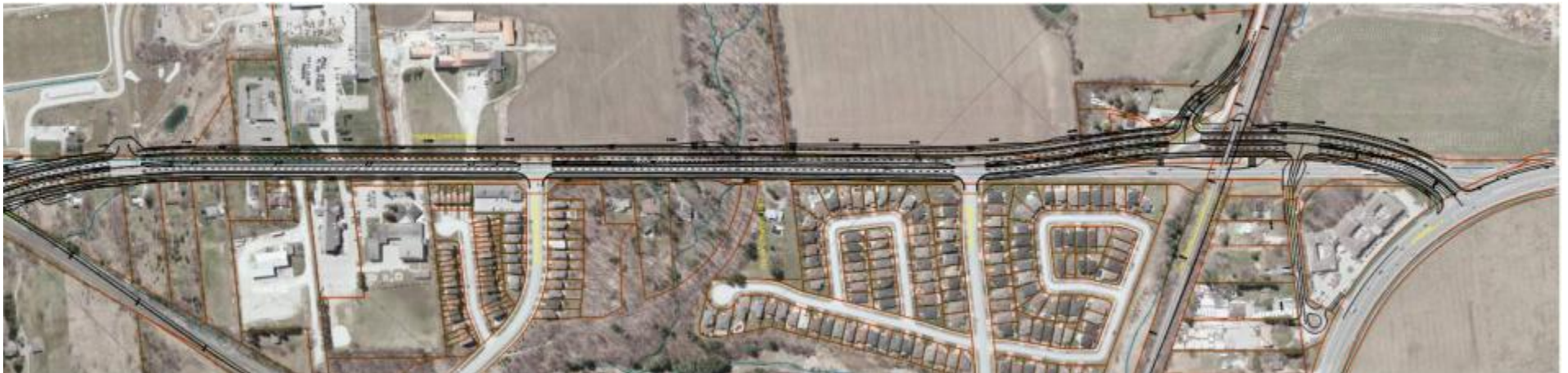
Trafalgar Road – north of CN Rail Crossing to Highway 7
