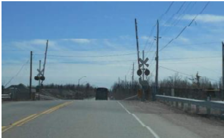
Existing At-Grade Metrolinx Crossing
