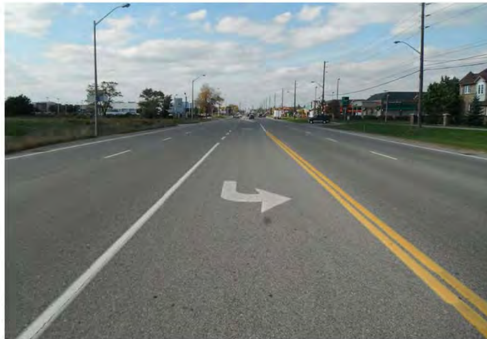
PHOTOGRAPH 6. Trafalgar Road, Section 2, showing pavement in fairly good condition.
