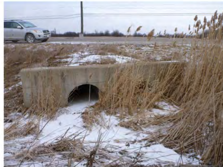
Photograph 8. East Morrison Creek – East Tributary C4 ↑ Channel is choked with vegetation on west side of culvert and exhibits a wide and shallow form. Definition increases in the downstream direction.
