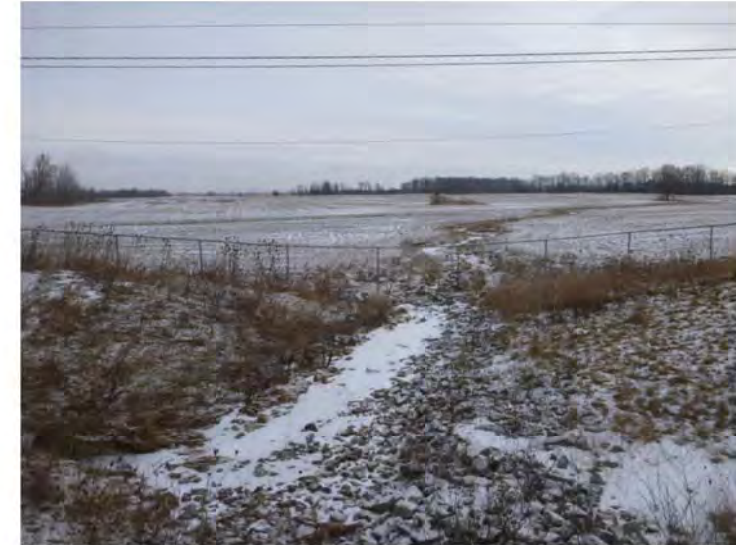
Photograph 1. Joshua Creek Crossing C1. ↑ Downstream of Trafalgar Road. The channel exhibits bank scour within the agricultural field
