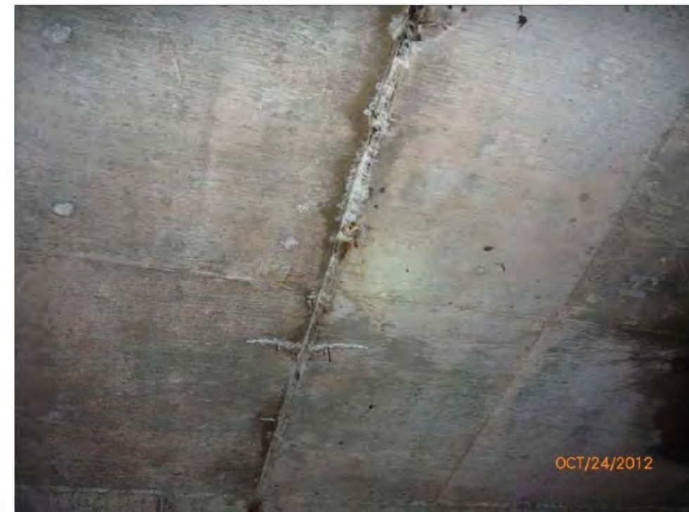
North Construction Joint
