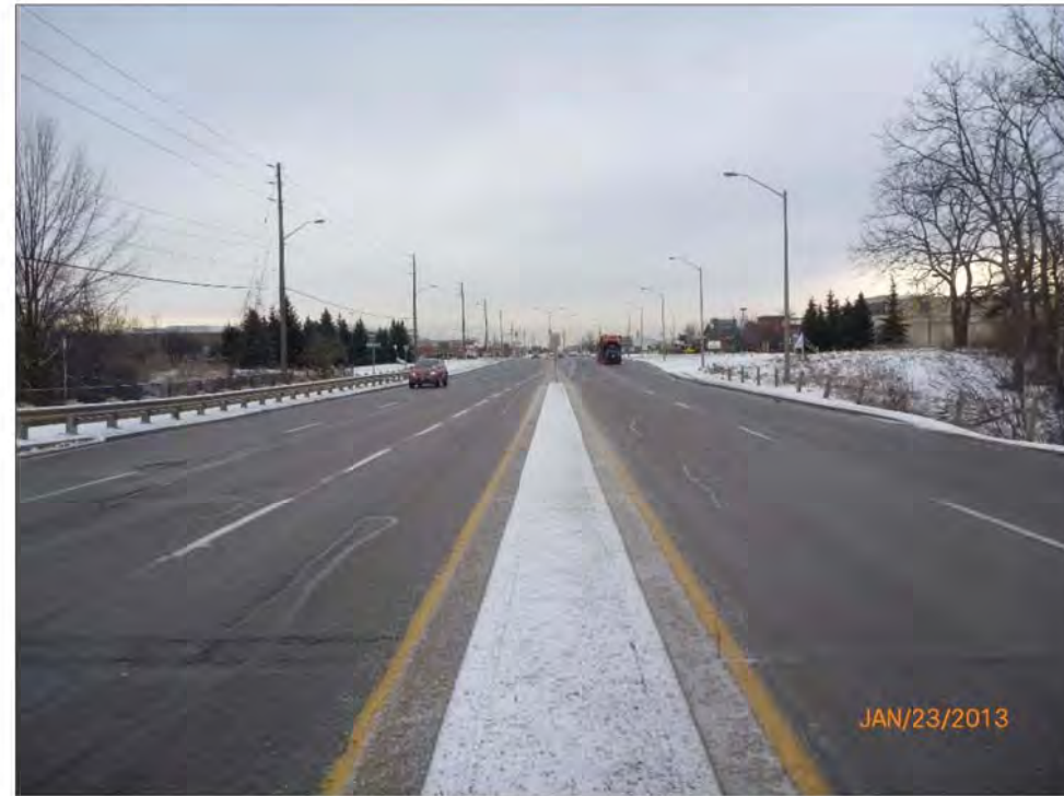
Looking South at Roadway Over Culvert
