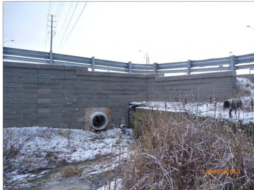
Typical Concrete Retaining Wall (East Side)
