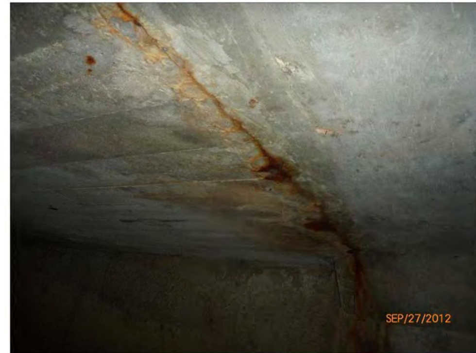
East Construction Joint
