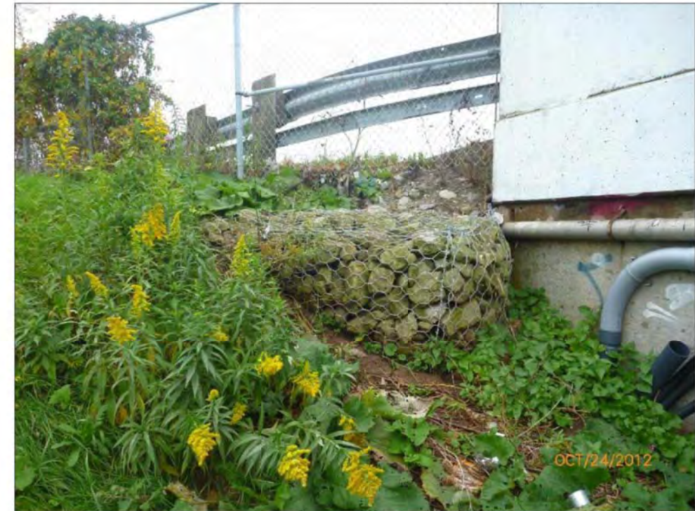
Typical Gabion Basket at East Side of Structure
