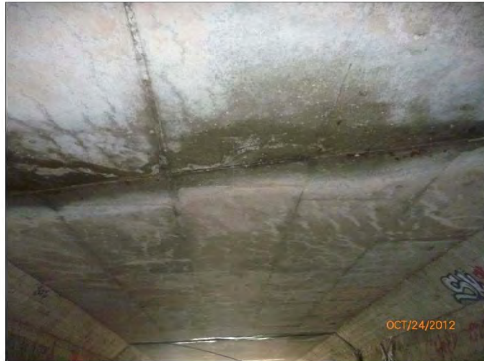
Middle Construction Joint
