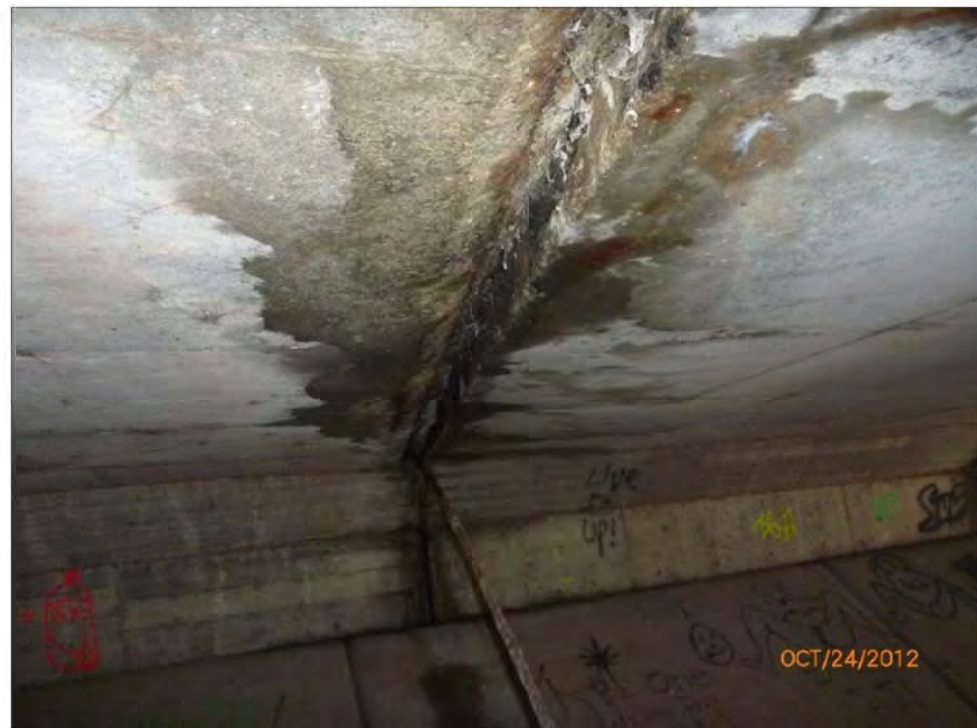
West Construction Joint
