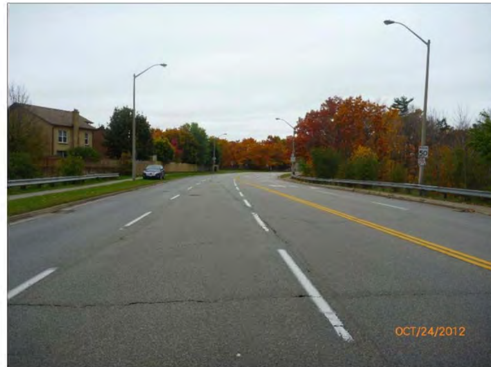
Looking West at Roadway Over Culvert
