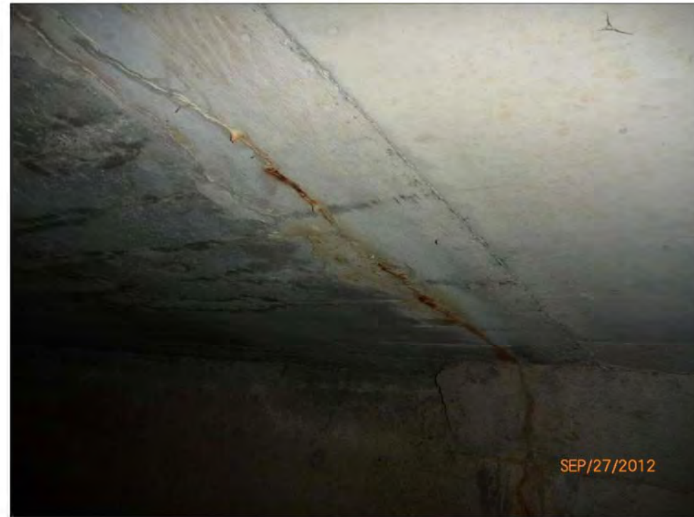
West Construction Joint
