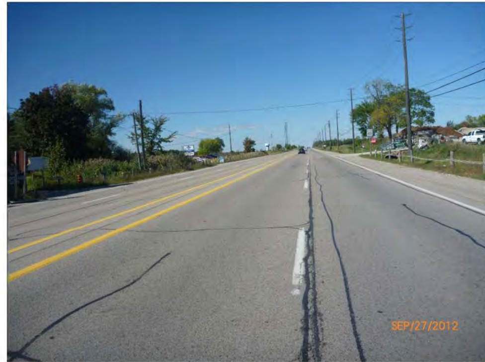
Looking North at Roadway Over Culvert
