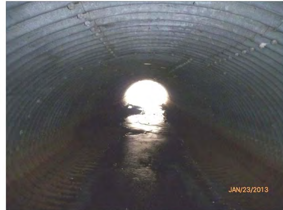
Looking West From Midspan
