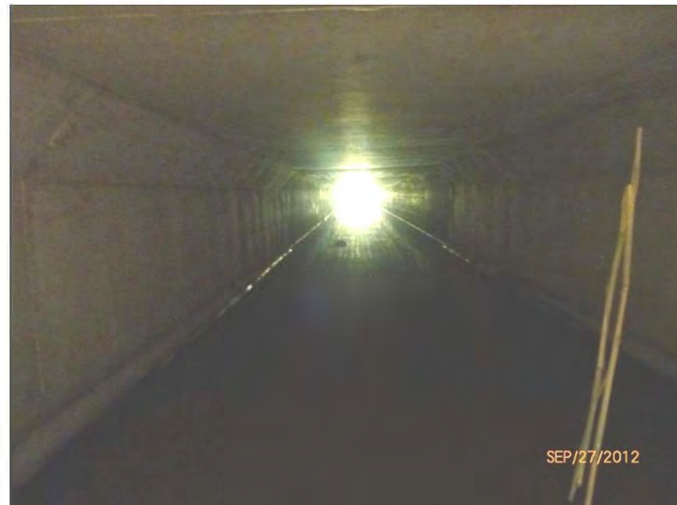
Looking East Through Barrel
