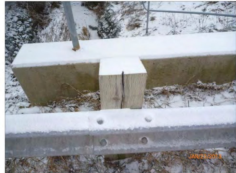
Checking of Flex Beam Wood Post
