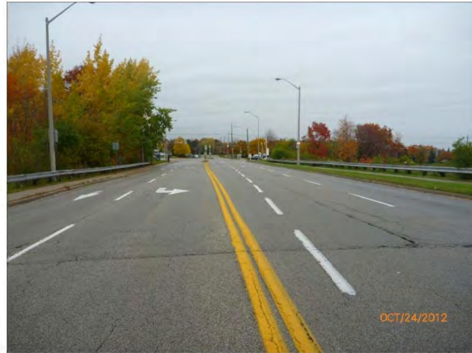
Looking East at Roadway Over Culvert
