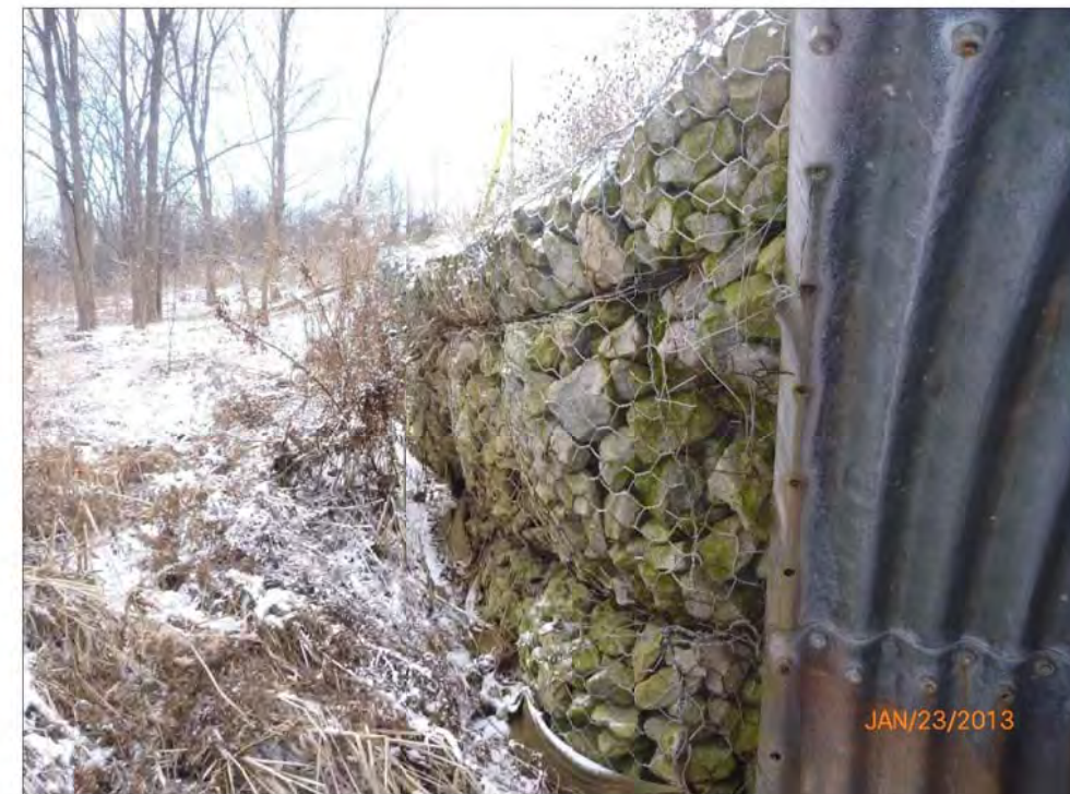
Minor Outward Rotation of Inlet Component
