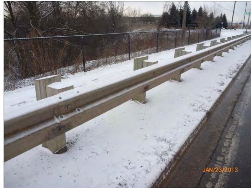
Typical Steel Flex Beam (East Side)
