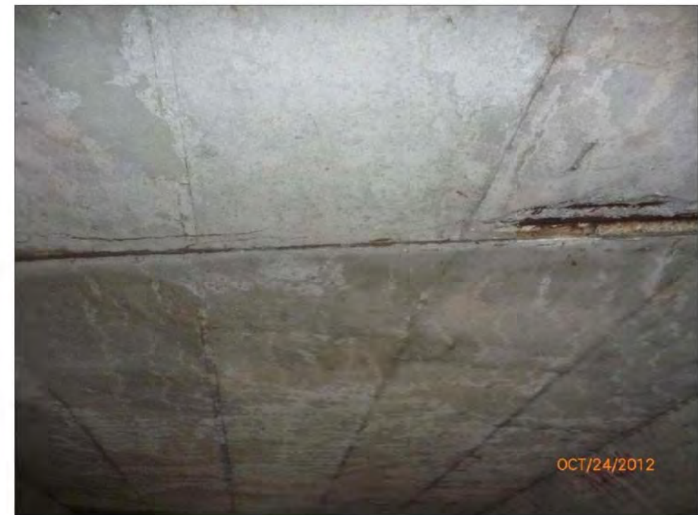
East Construction Joint
