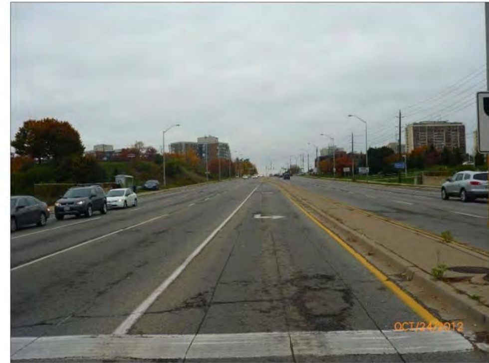
Looking North at Bridge
