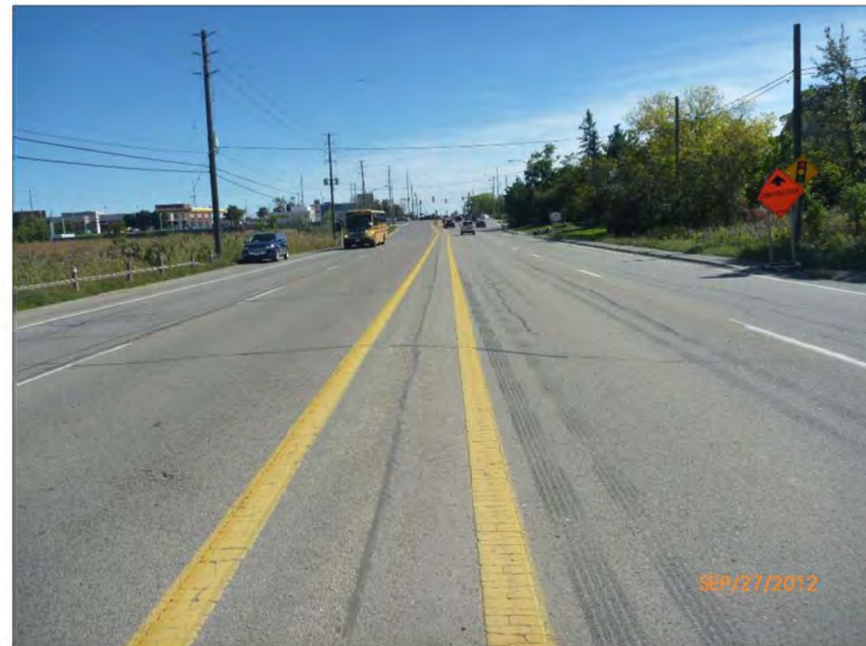
Looking South at Roadway Over Culvert
