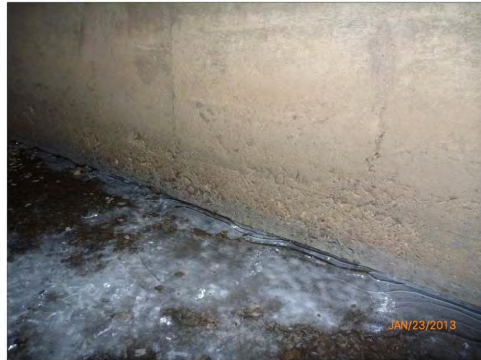
Light Scaling of Original Barrel Wall
