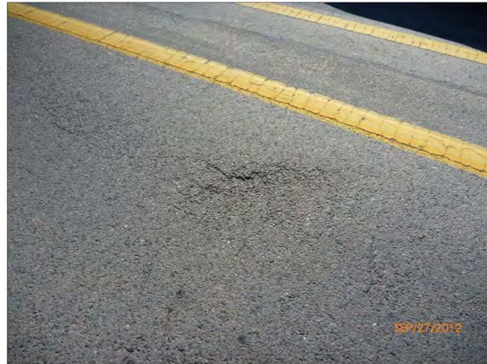
Medium Ravelling on Wearing Surface
