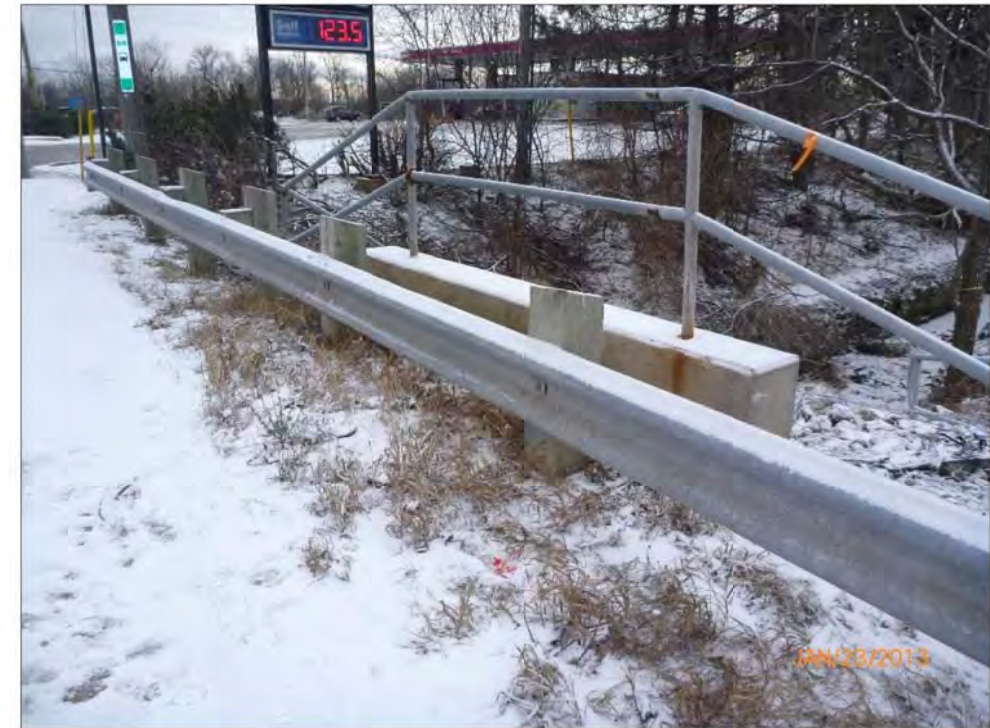
Typical Steel Flex Beam (West Side)
