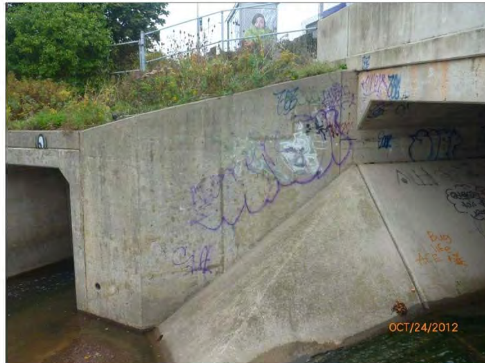
Typical Retaining Wall in Northwest Quadrant
