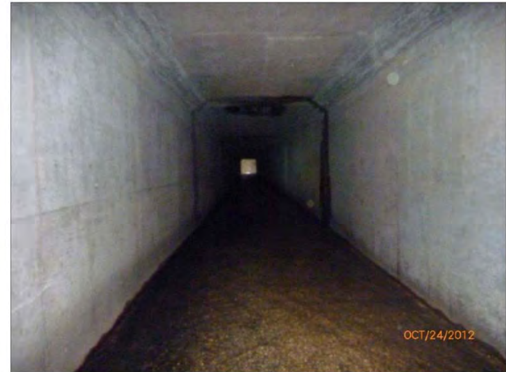
Looking South Through Barrel at Midspan
