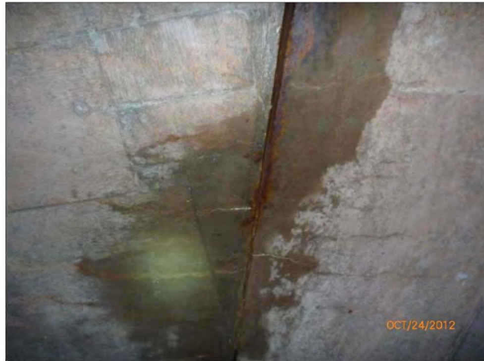
South Construction Joint
