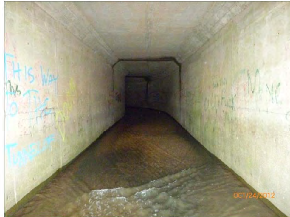
Looking North Through Barrel
