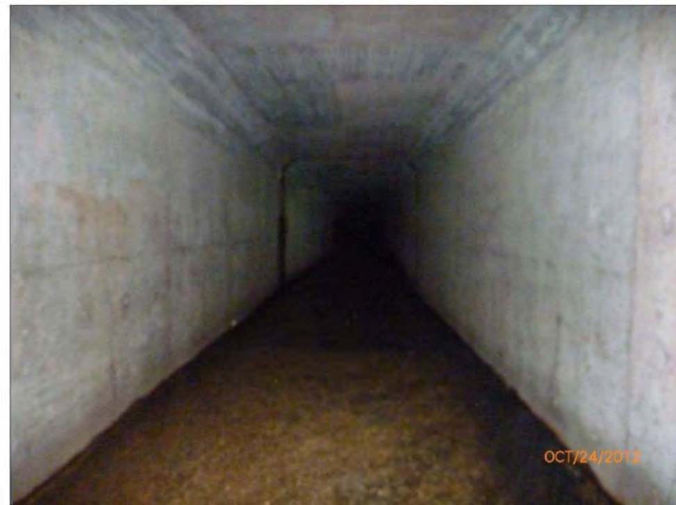
Looking North Through Barrel at Midspan
