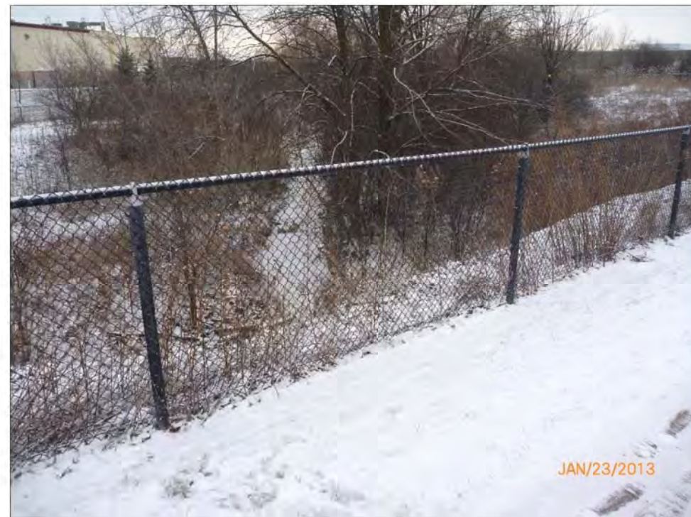
Typical Chain Link Fence (East Side)
