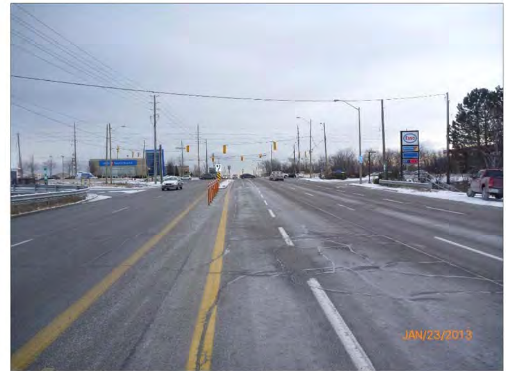
Looking South at Roadway Over Culvert
