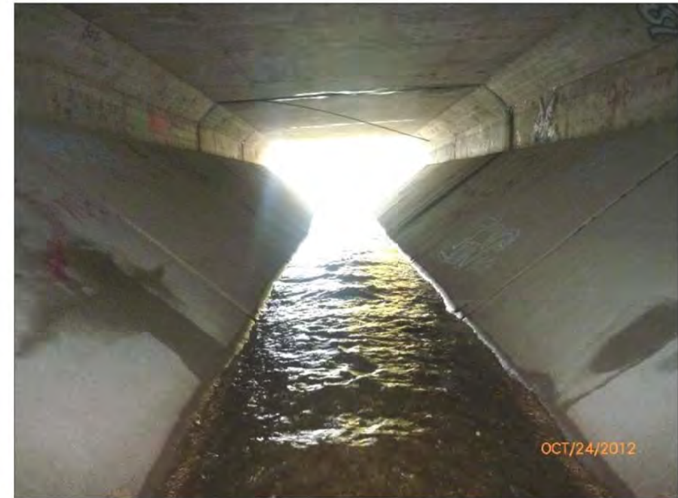
Watercourse Below Structure
