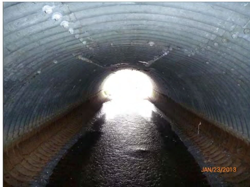
Looking East From Midspan
