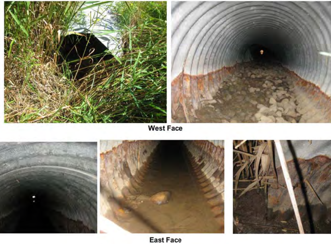
East Face Figure 2.9 Culvert 6+200 (ME-T4)
