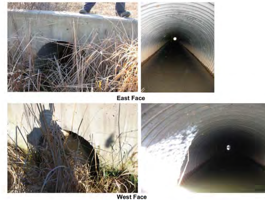
West Face Figure 2.10 Culvert 5+820 (ME-T3) (North Cell)
