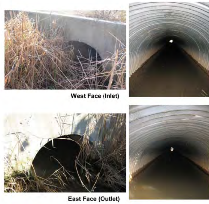
Figure 2.11 Culvert 5+820 (ME-T3) (South Cell)
