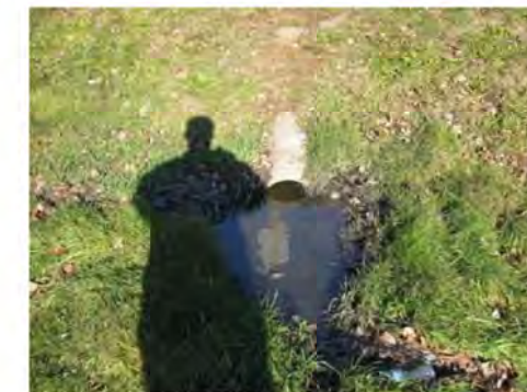
Figure 2.1 Trafalgar Road West Side Storm Sewer Outlet to Ditch
