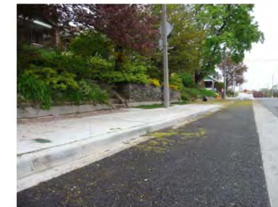
Figure 3.8 Permeable Asphalt Parking
