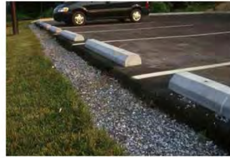
Figure 3.3 Pea Gravel Diaphragm Applied as Level Spreader for Parking Lot Runoff
