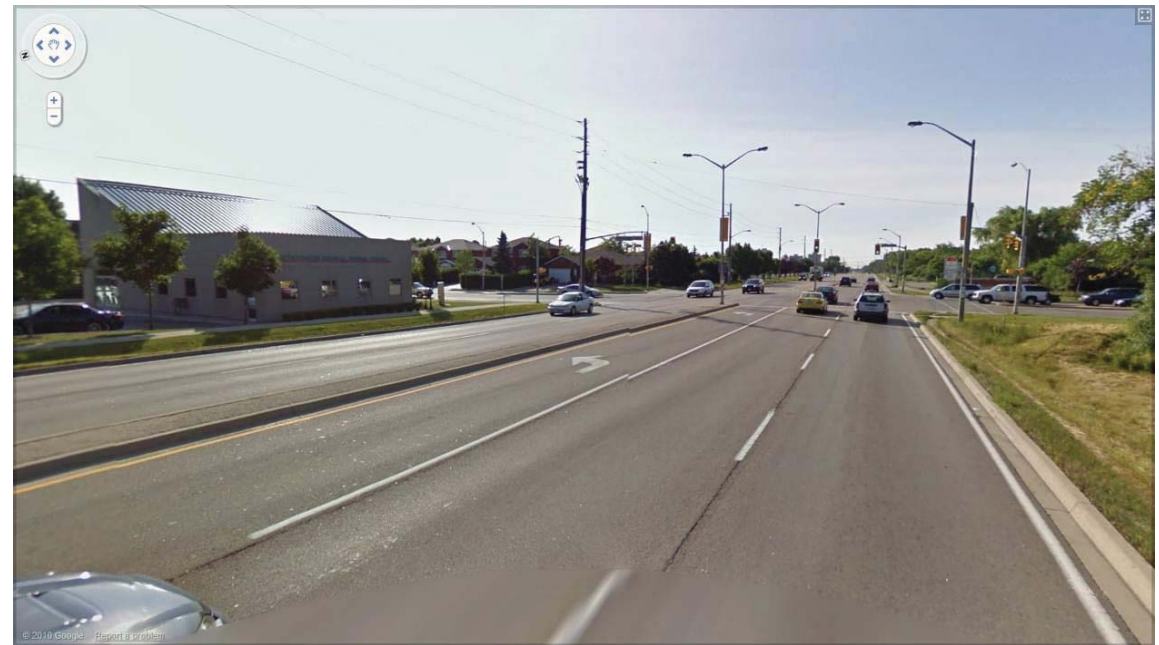
Image 2: Looking slightly southeast along Trafalgar Road at paved roadway and narrow shoulder, ditching, utilities, paved sidewalks, and landscaping
