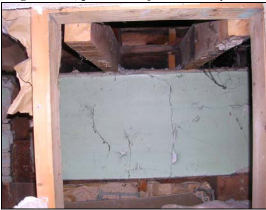
Cut ceiling joists of original building.
