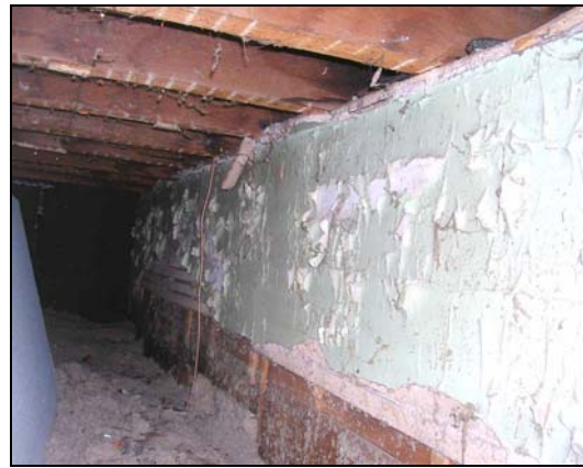
View of lath markings of schoolhouse ceiling on joists.
