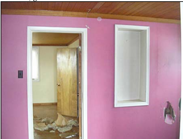
Hallway 2 nd floor.
