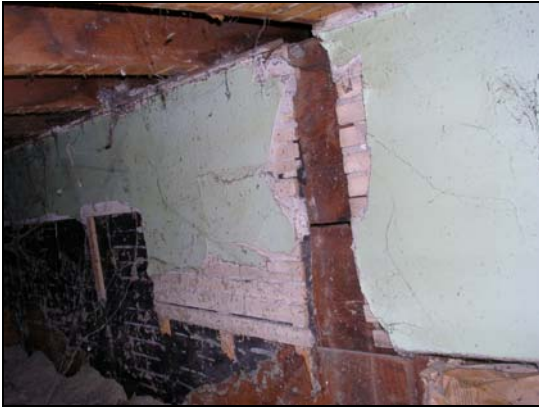
Original wall, plaster and joist assembly.
