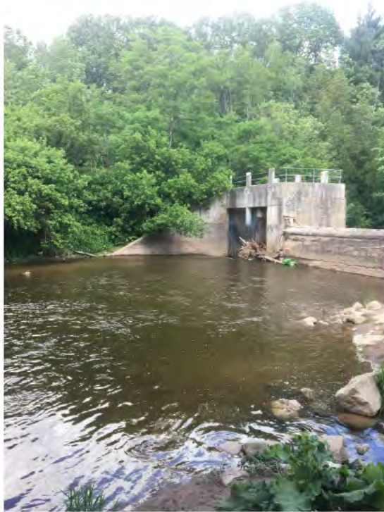
Photo 3: Paper Mill Dam at downstream end of Study Area
