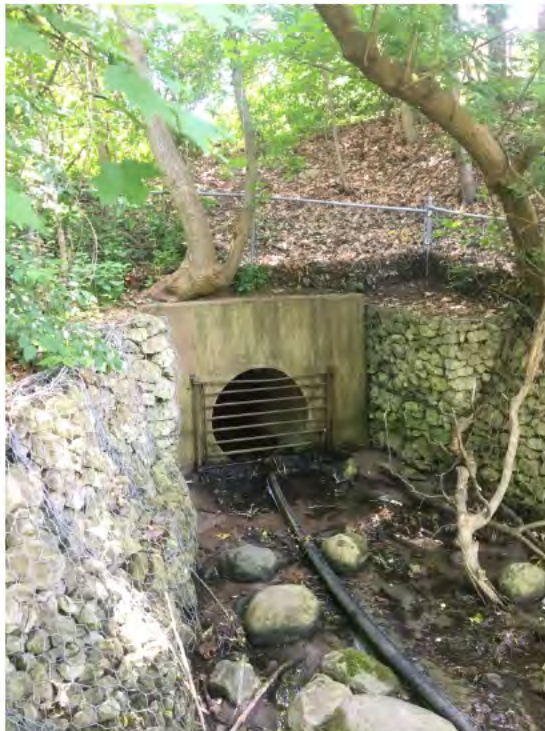
Photo 4: Stormwater outlet between Pond 1 and Pond 2
