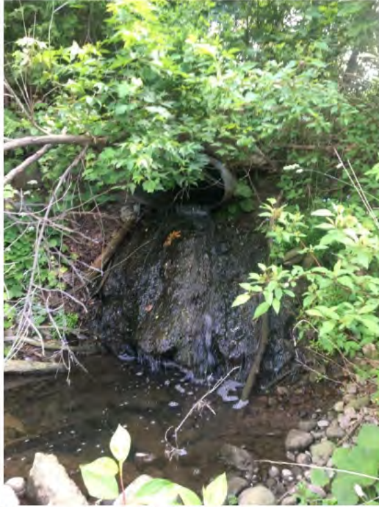
Photo 5: Stormwater discharge to Credit River
