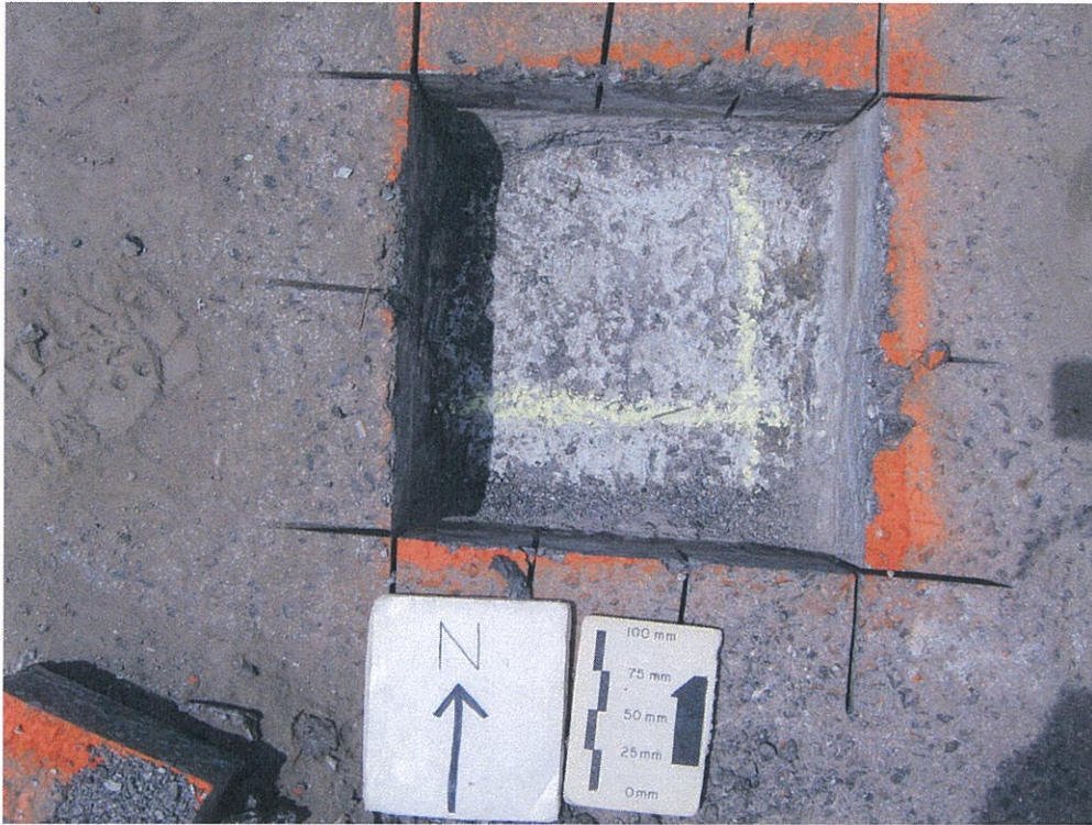
Sawn Asphalt S1
