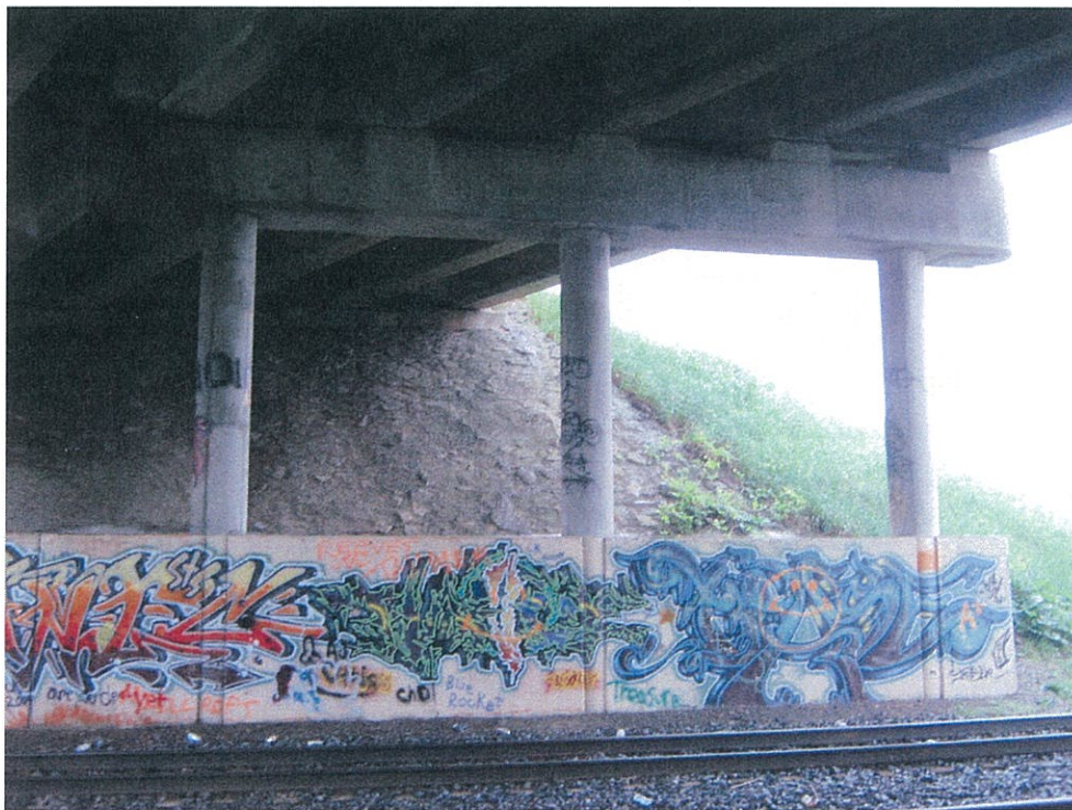
Photograph 4 – Northwest pier, looking west
