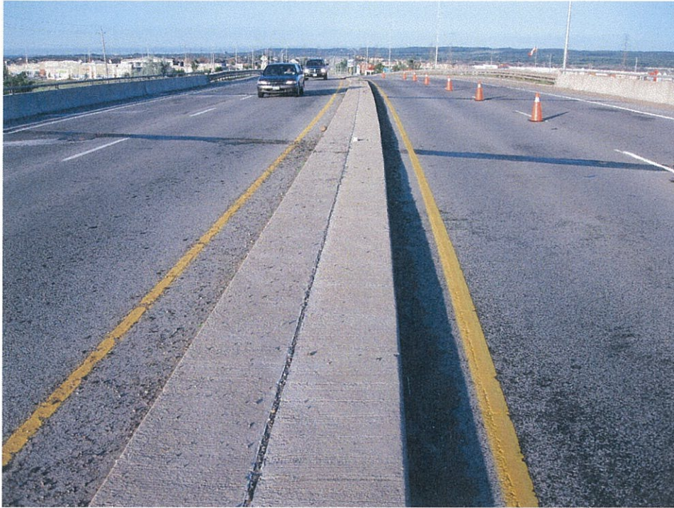
Photograph 7 – West approach, looking west
