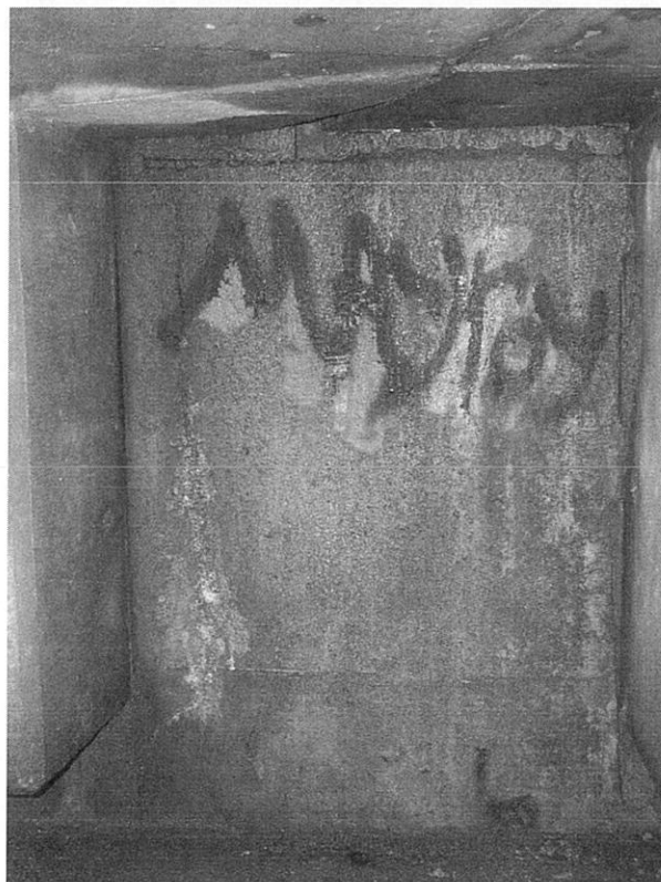
Photo 5 – East Abutment below the Longitudinal Expansion Joint
