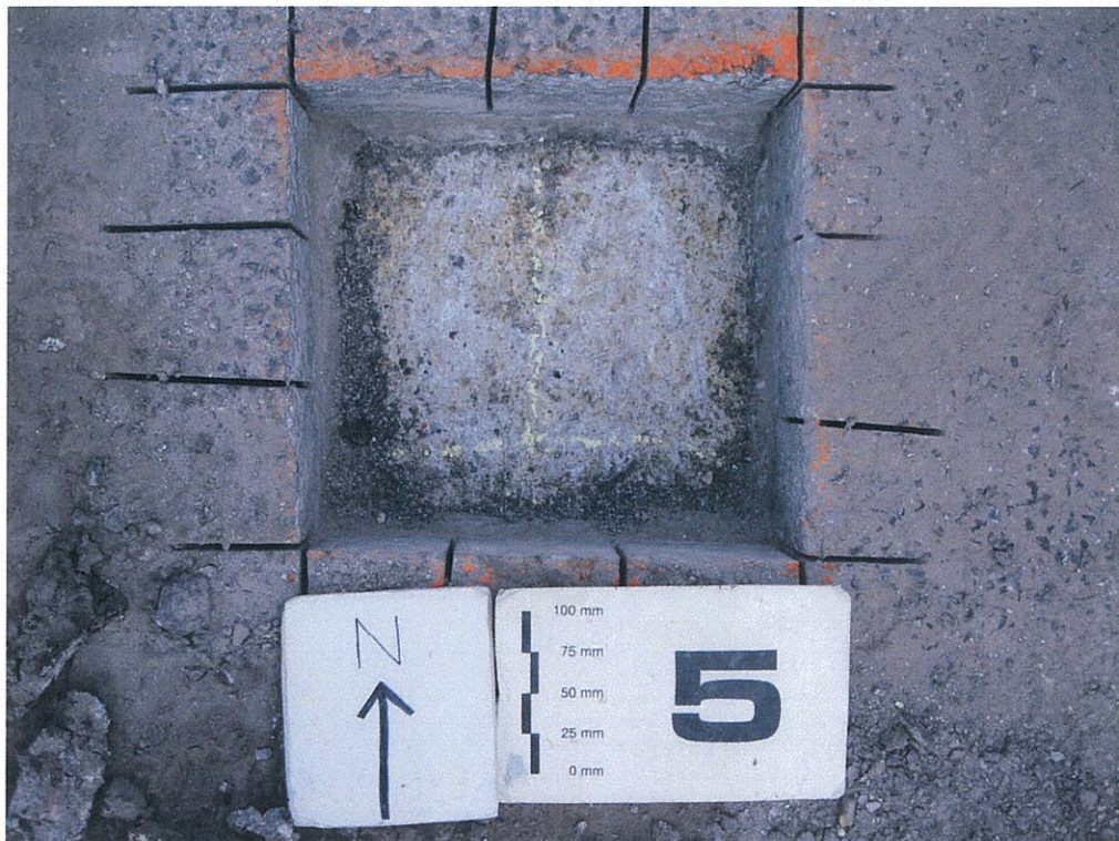
Sawn Asphalt S5
