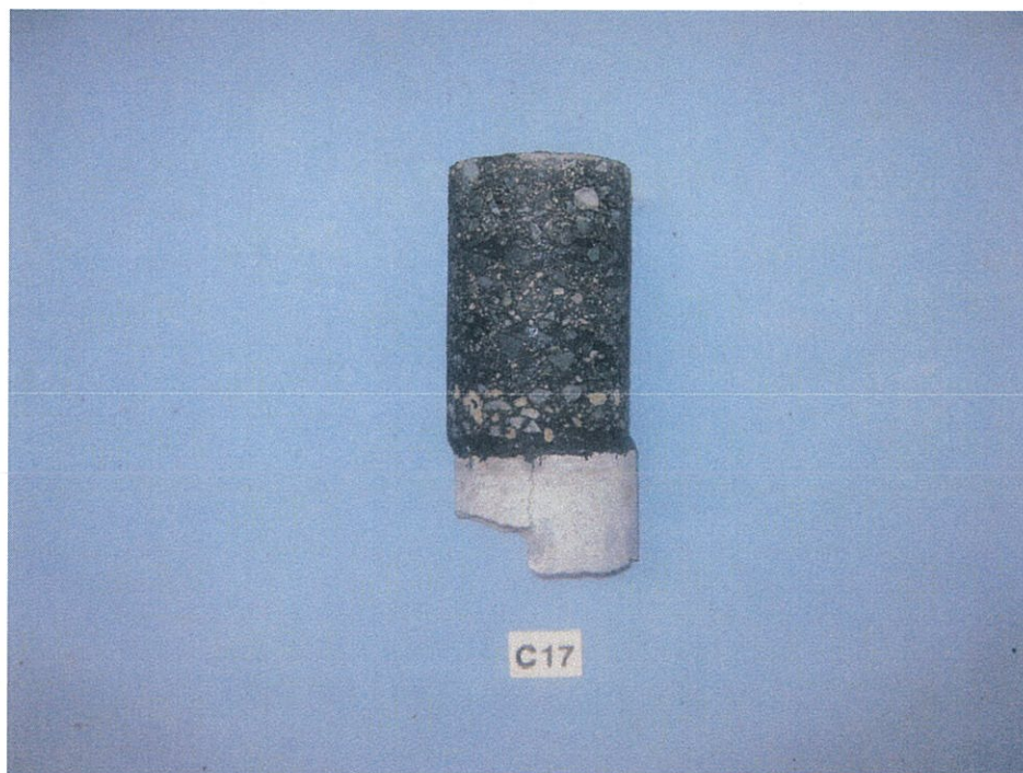
Photograph 16 – Vertical crack in core C17
