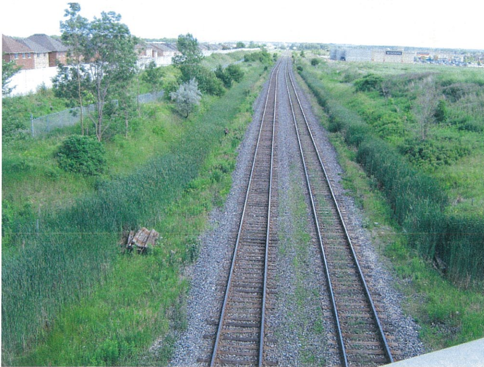
Photograph 8 – Looking south along CN rails
