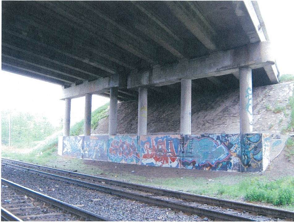
Photograph 5 – East piers, looking northeast
