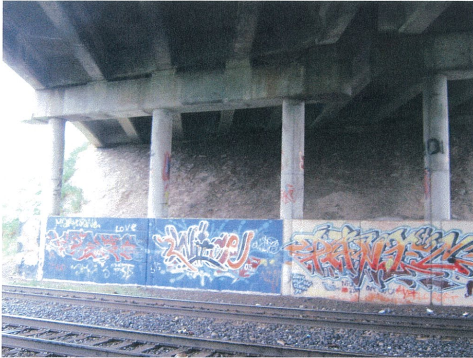
Photograph 3 – Southwest pier, looking west
