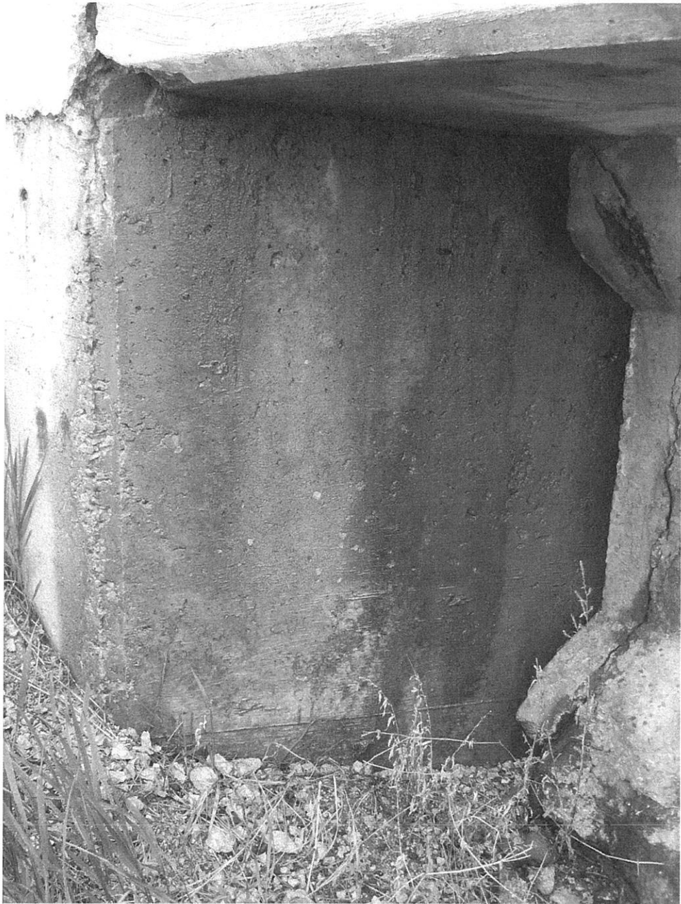
Photo 3 – South Girder at West Abutment
