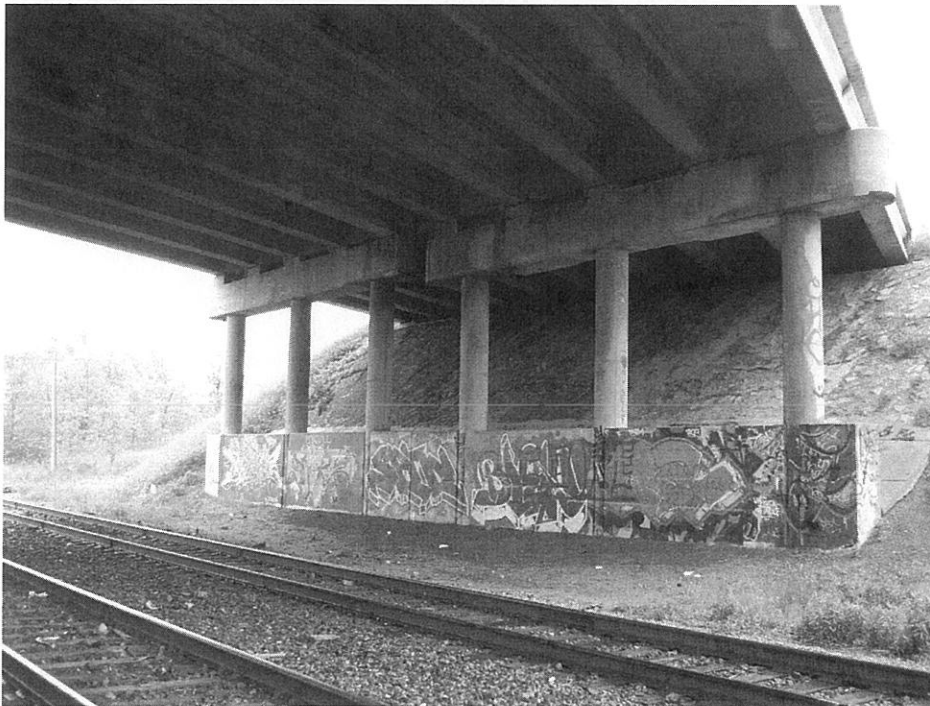
Photo 7 – Vegetation at Slope Paving
