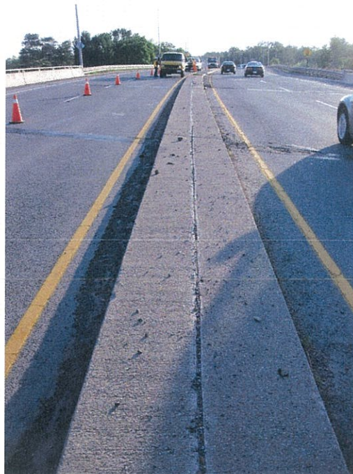
Photograph 18 – Longitudinal joint along the raised median (installed during 2004 rehabilitation contract)
