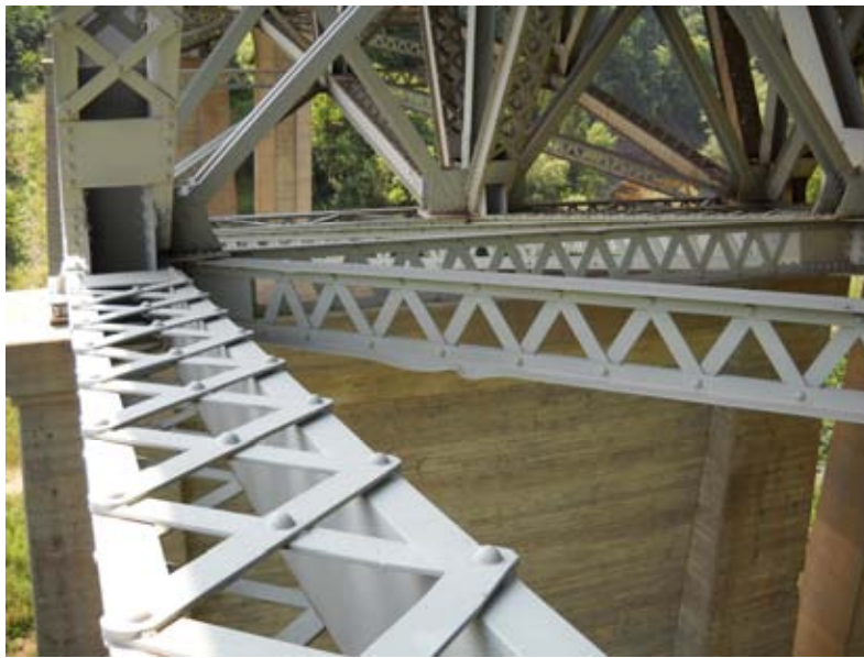
TRUSS SUPERSTRUCTURE: BOTTOM CHORD AND BRACING
