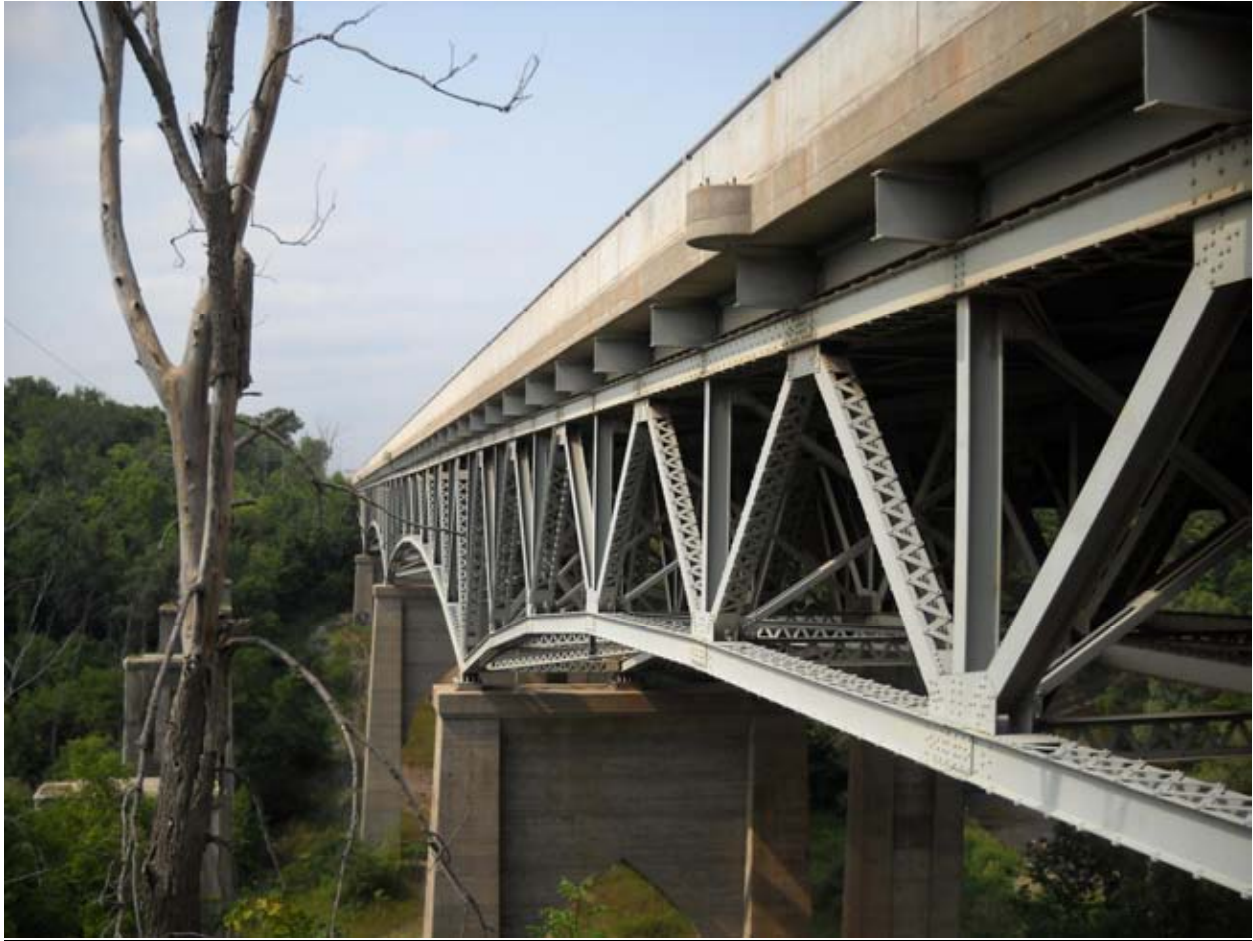
TRUSS BRIDGE: ELEVATION VIEW
