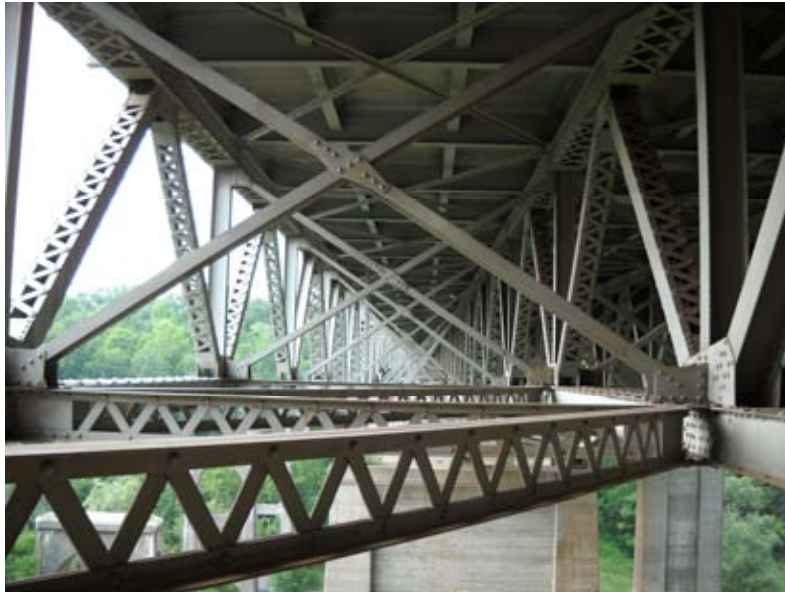
TRUSS SUPERSTRUCTURE: CROSS-FRAMES
