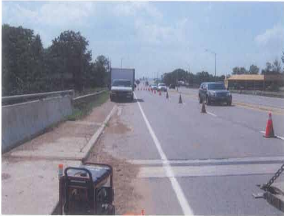
Photograph 3. West approach, looking west from bridge
