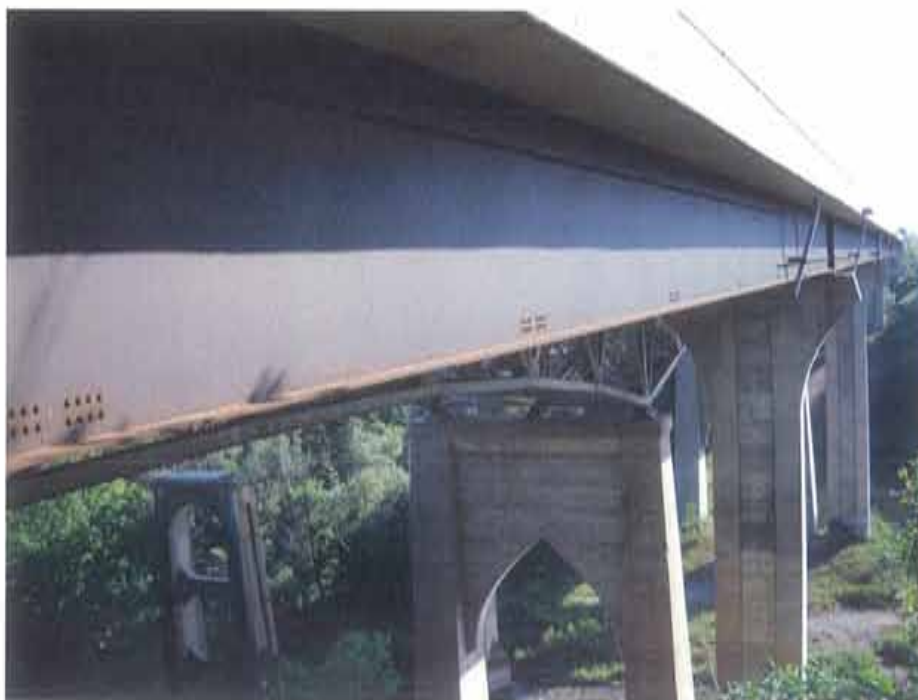
Photograph 2. North elevation of north structure
