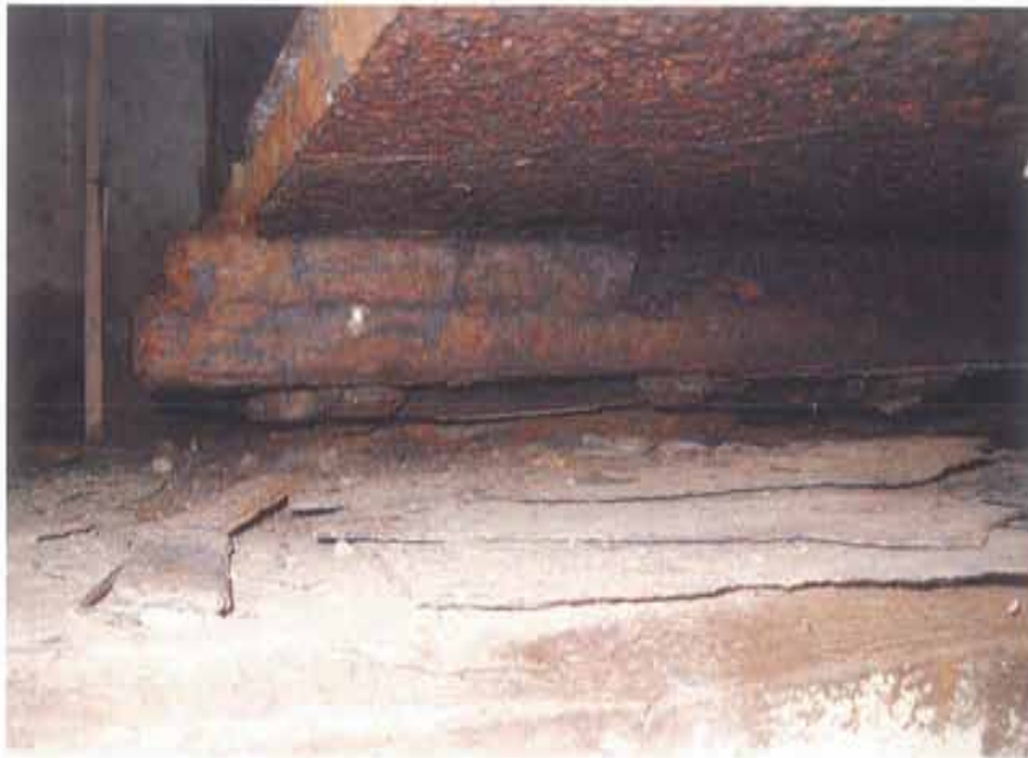
Photograph 91. Typical condition of bearings at west abutment, G3 shown
