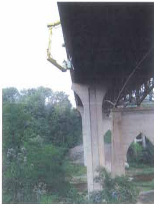
Photograph 44. MRC inspection crew inspecting girder 'G1' of the south structure
