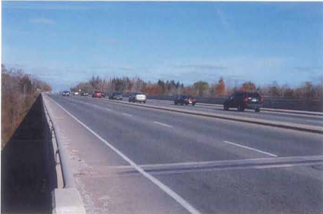
Photograph 8. General view of the bridge deck, looking southeast
