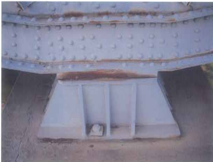
Photograph 76. Typical fixed pier bearing condition, T3/L28 shown at the centre pier
