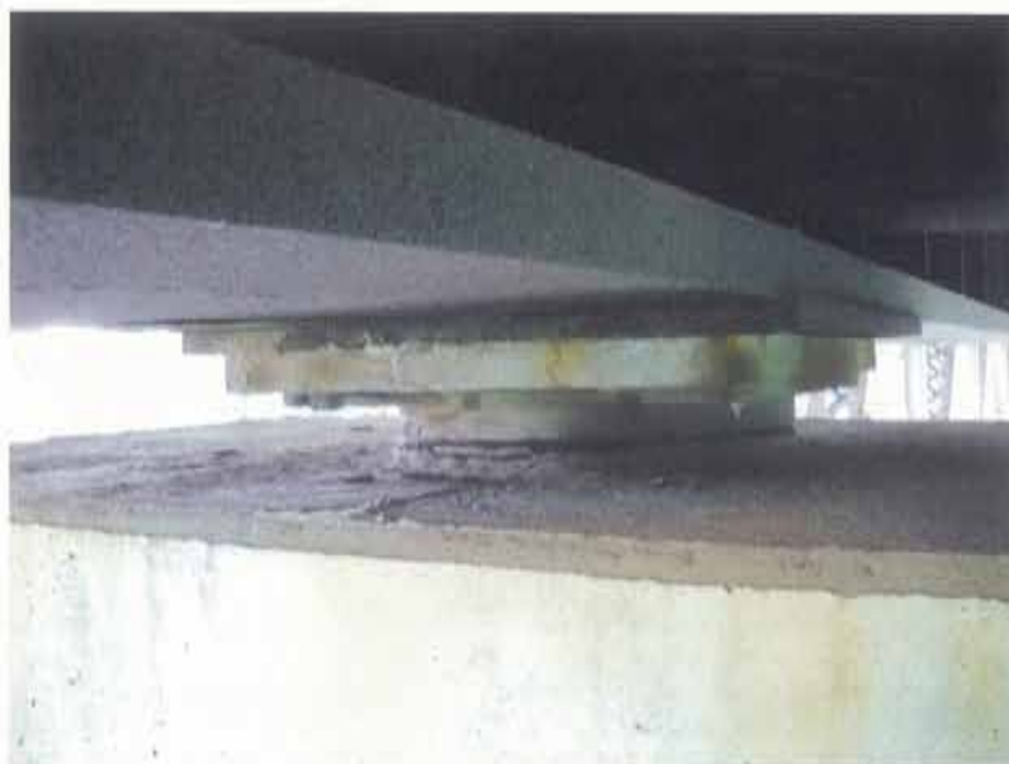
Photograph 90. Typical condition of bearings at east pier, G3 shown
