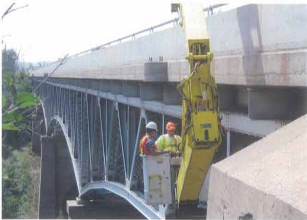
Photograph 1. South elevation of south structure
