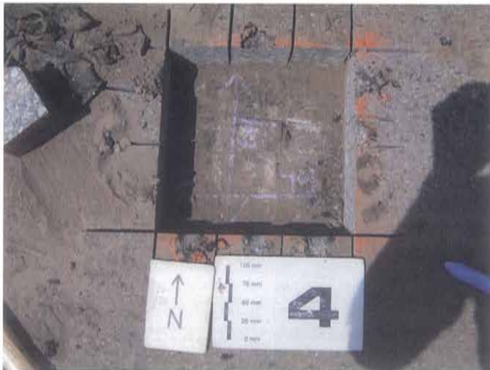
Sawn Asphalt S4
