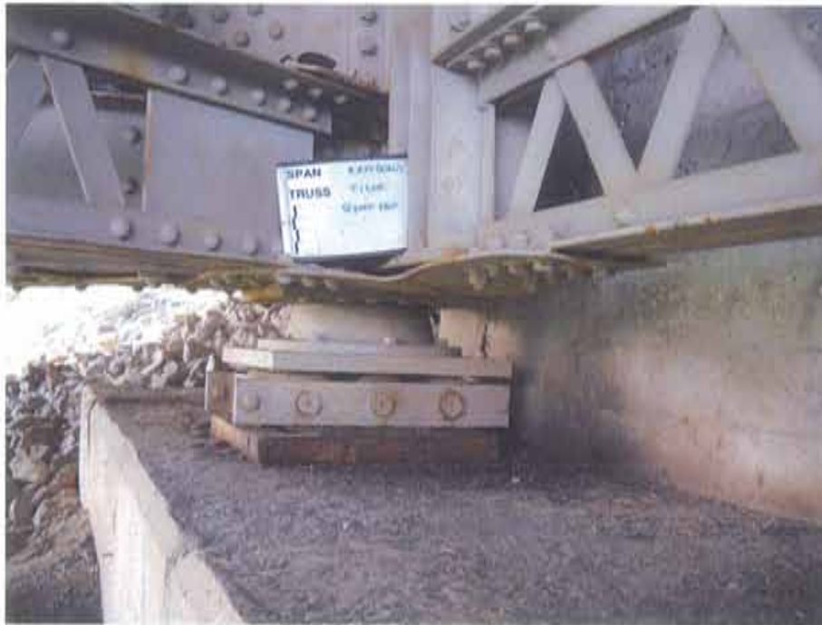
Photograph 75. Typical abutment bearing condition, T1/L0E shown at east abutment
