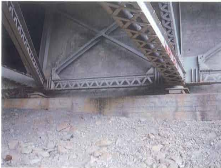
Photograph 65. East abutment of north structure (T1 and T2 shown)
