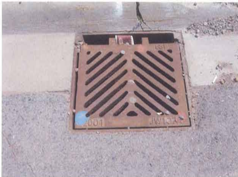
Photograph 20. Typical catch basin west of bridge existing on both the north and south structures
