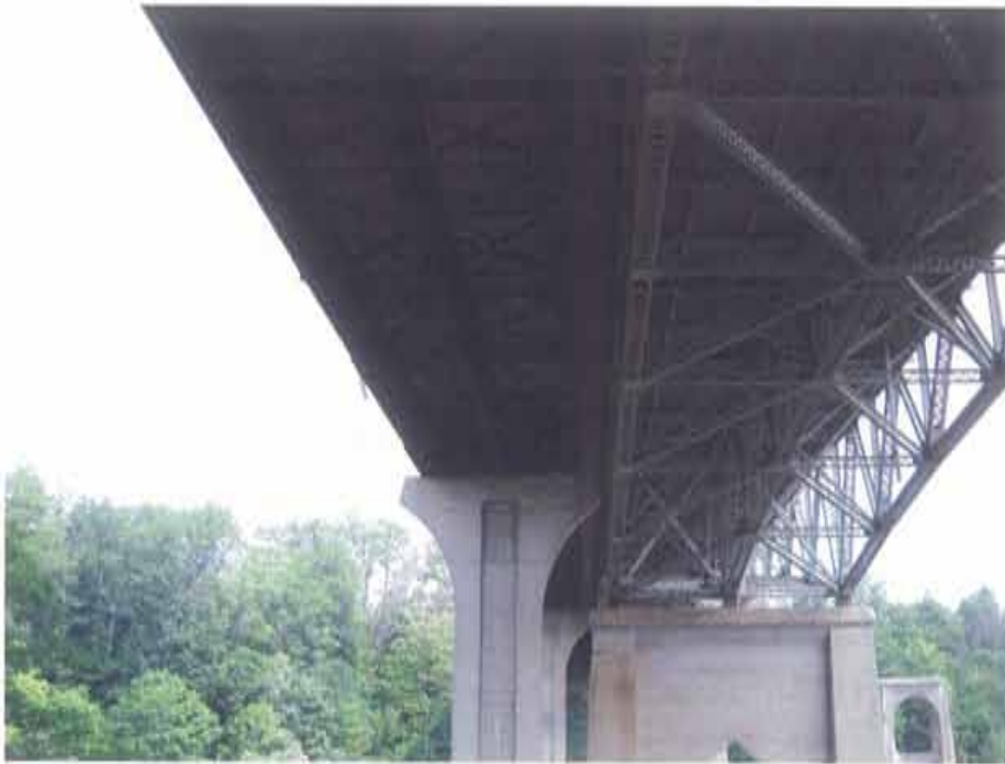
Photograph 7. Underside of bridge, looking east (west interior span shown)
