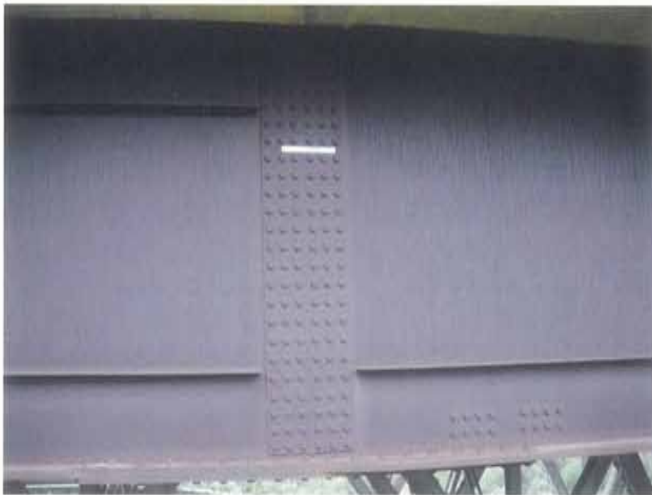
Photograph 78. Web splice plate, G1 shown
