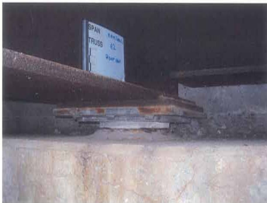
Photograph 89. Typical condition of bearings at east abutment, G2 shown
