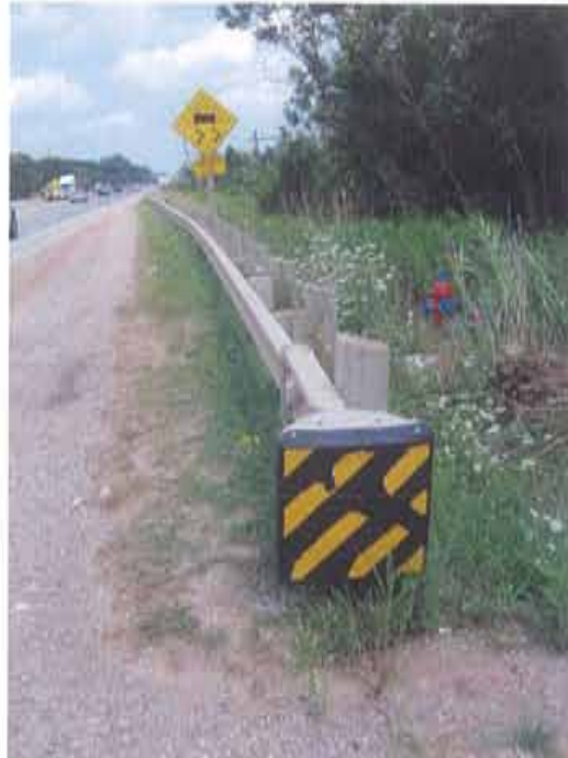
Photograph 32. Southwest steel beam guiderail with crash attenuator, looking east (typical); note: the fire hydrant
