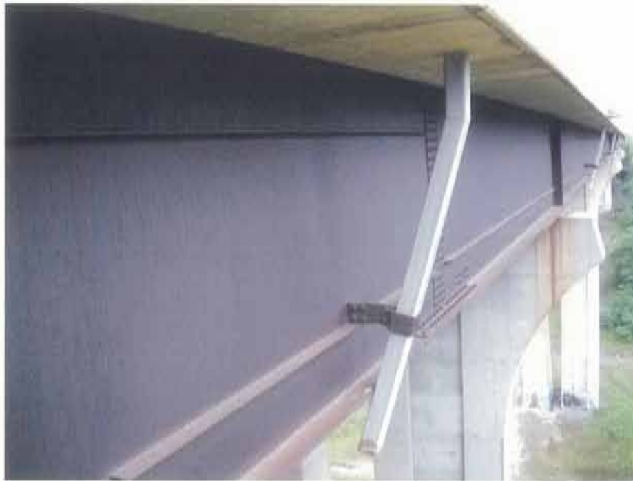
Photograph 77. Typical condition of G1, east exterior span shown
