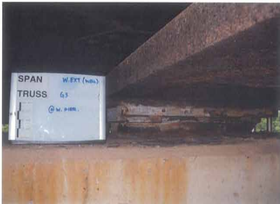
Photograph 92. Condition of bearing supporting G3 at the west pier
