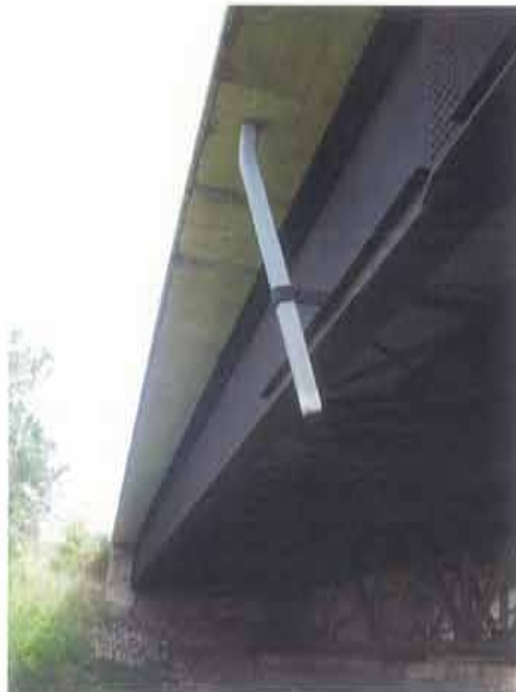
Photograph 80. East abutment of north structure
