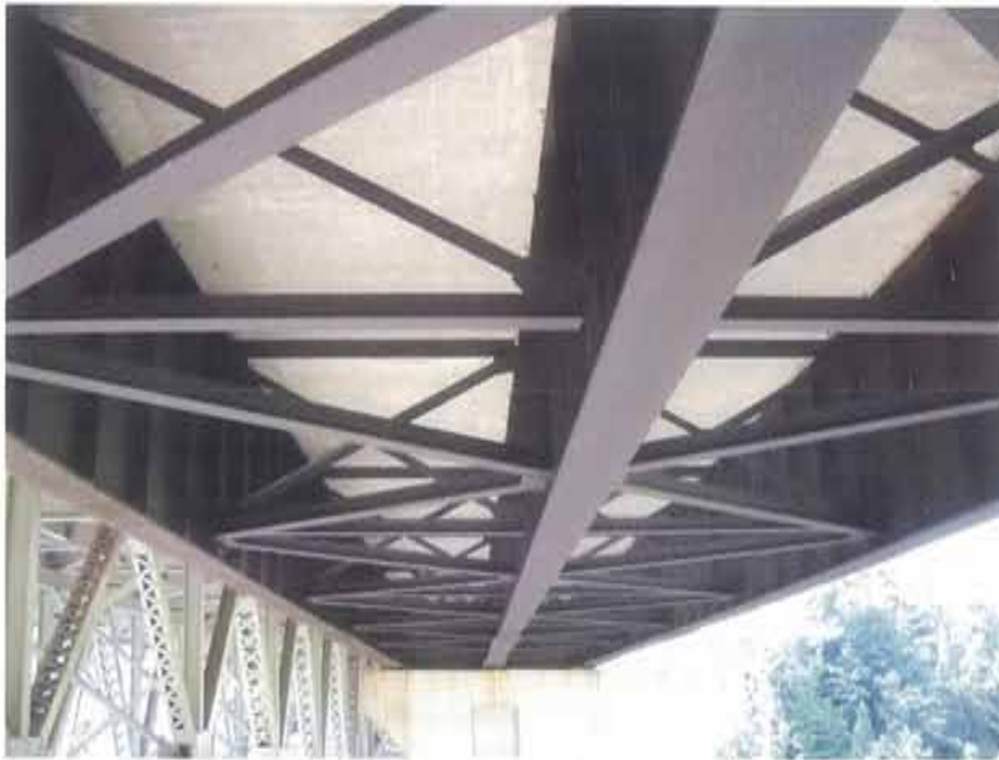
Photograph 79. Underside of north structure, east interior span shown
