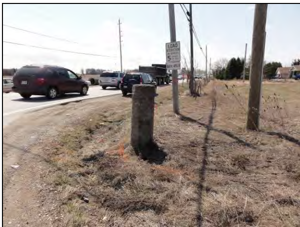
Plate 3: Example of a plain, cylindrical poured concrete corner fence post.
