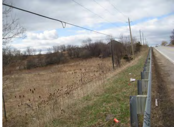
Plate 12: South view from Britannia Rd of valley bottom and road fill.
