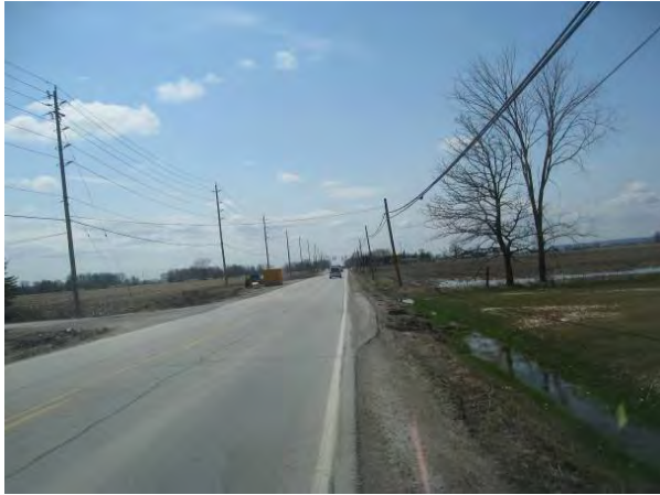
Plate 31: Southwest view along Britannia Rd. Disturbed ROW and wet land with no potential. Field beyond wet land has potential.
