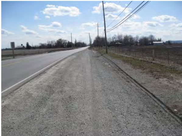
Plate 27: Southwest view along Britannia Rd. Disturbed ROW with no potential.
