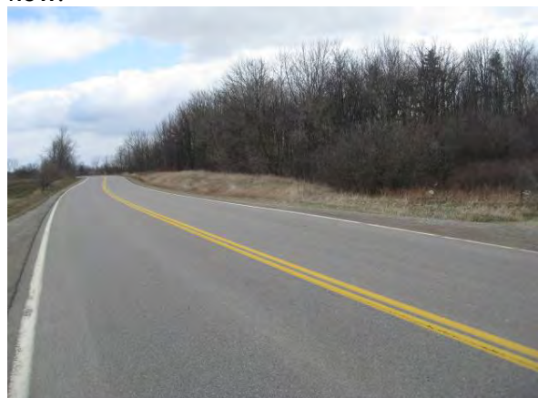
Plate 6: Northeast view along Britannia Rd. Disturbed ROW. Wet on both sides of road.
