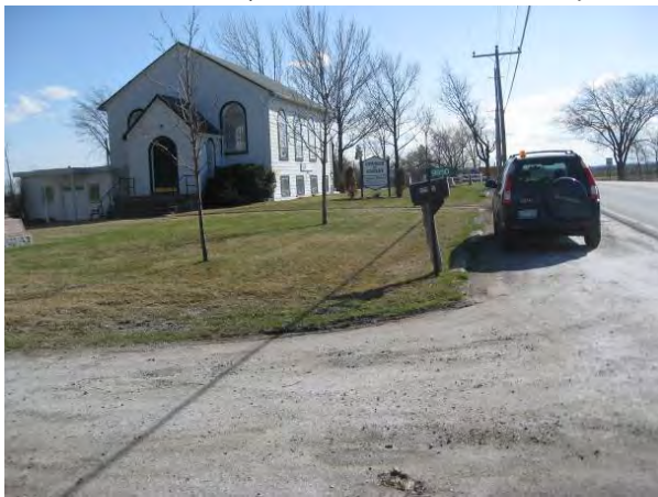
Plate 21: Southwest view of church and cemetery grounds. ROW in front of cemetery requires Cemetery Investigation.
