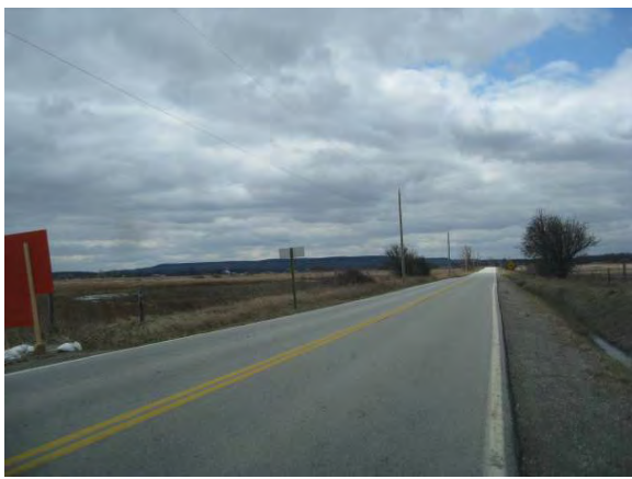
Plate 5: South view across Britannia Rd. Disturbed ROW with no potential. Potential on both sides of road in fields.
