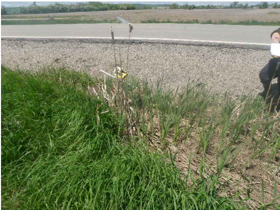
Crossing 4 – Downstream facing culvert
