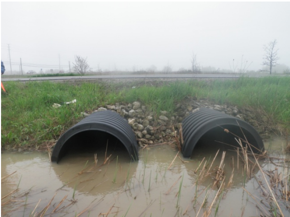
Crossing 6 – Upstream facing culvert
