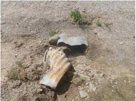
Crossing 13 – Downstream facing culvert
