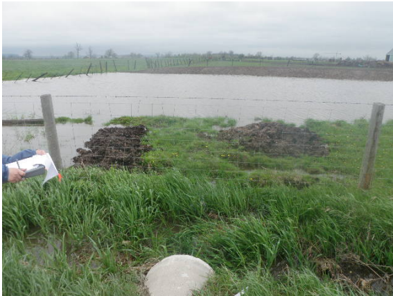
Crossing 10 – Looking upstream
