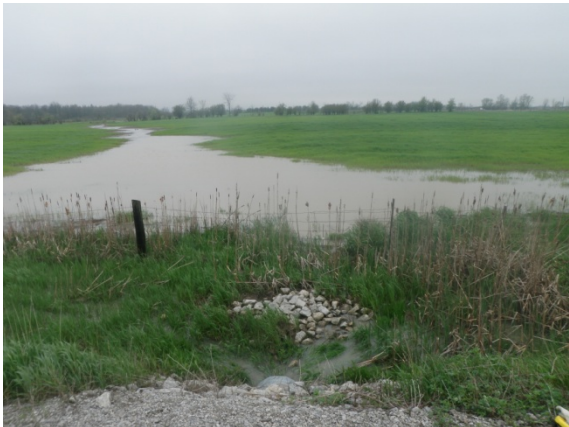
Crossing 8 – Looking upstream
