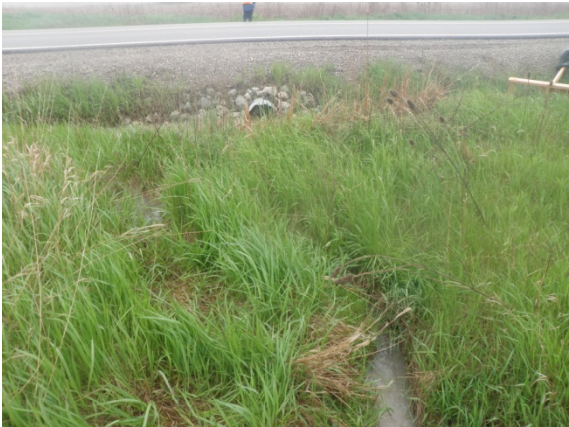
Crossing 5a – Looking downstream
