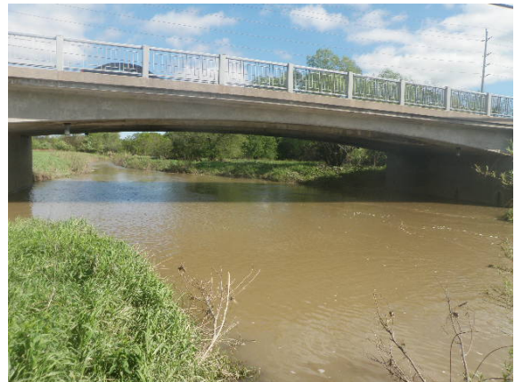
Crossing 15 – Upstream facing bridge
