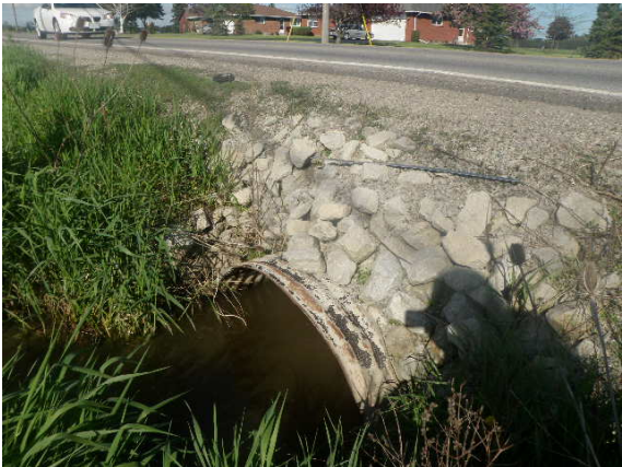
Crossing 16 – Upstream facing culvert
