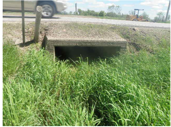
Crossing 14 – Upstream facing culvert
