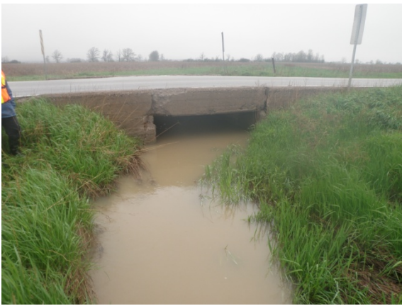
Crossing 1 – Downstream facing culvert
