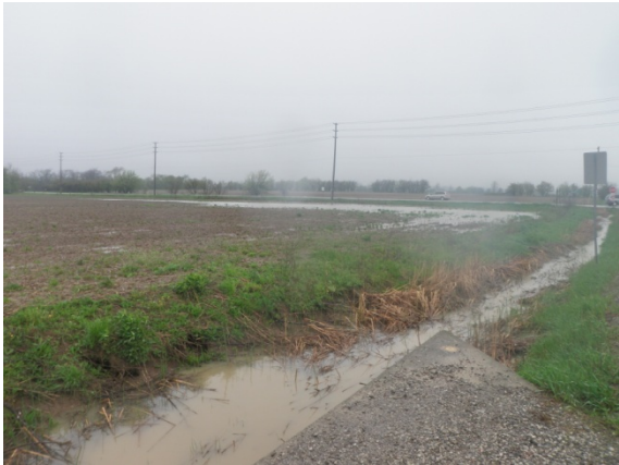
Crossing 3 – Looking upstream to the east
