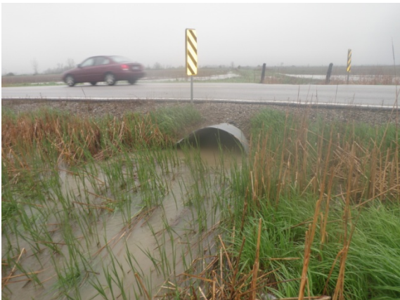
Crossing 2 – Downstream facing culvert
