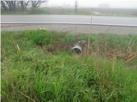
Crossing 5a – Upstream facing culvert
