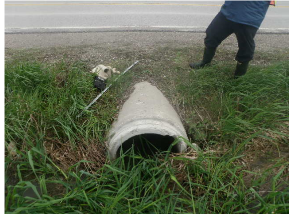
Crossing 10 – Upstream facing culvert
