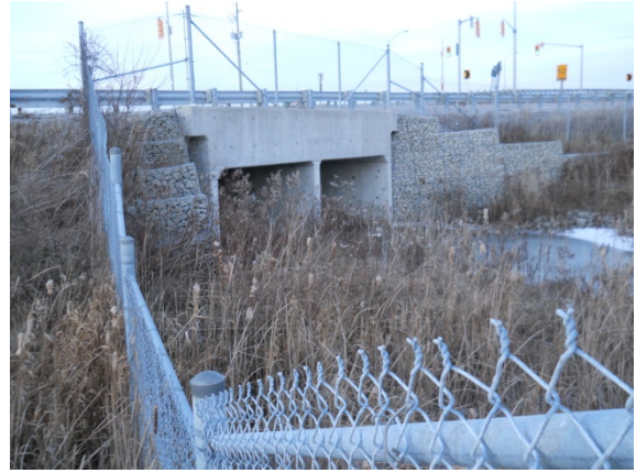
Crossing 18 – Downstream facing culvert
