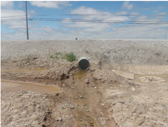
Crossing 12 – Downstream facing culvert
