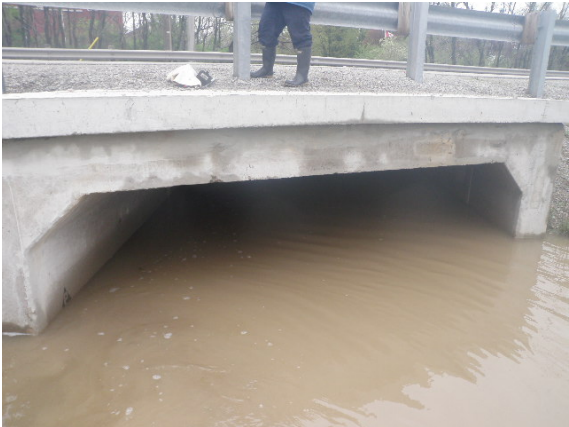
Crossing 9 – Upstream facing culvert
