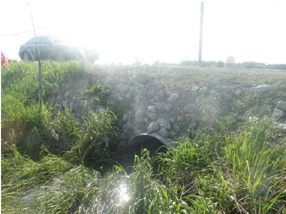
Crossing 17 – Downstream facing culvert
