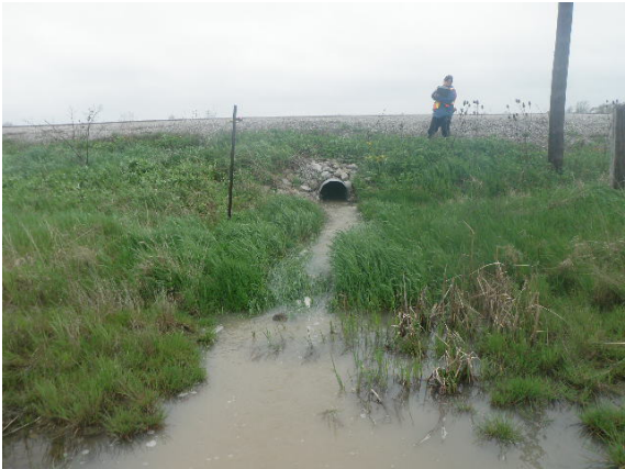
Crossing 8 – Downstream facing culvert
