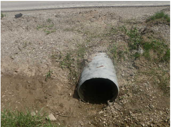
Crossing 13 – Upstream facing culvert
