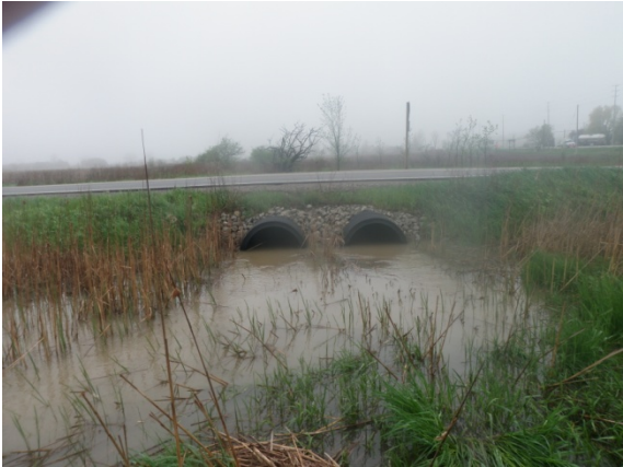
Crossing 5a – Downstream facing culvert
