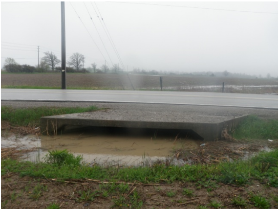
Crossing 3 – Upstream facing culvert
