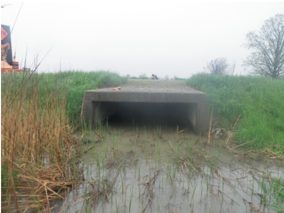
Crossing 5 – Downstream facing culvert
