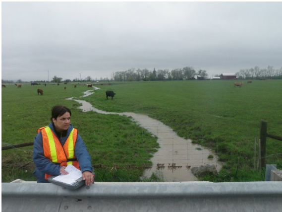
Crossing 9 – Looking upstream
