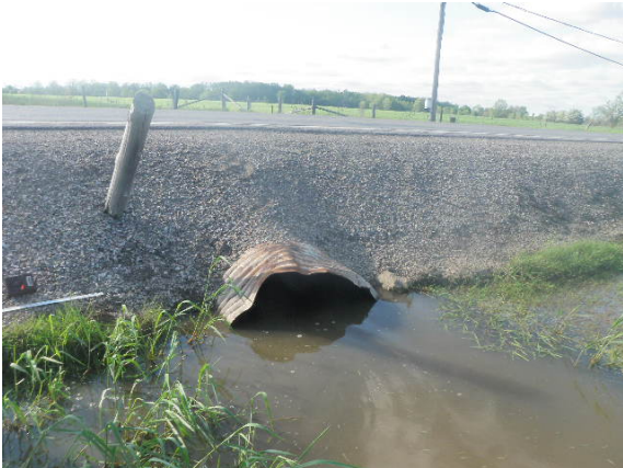
Crossing 16 – Downstream facing culvert
