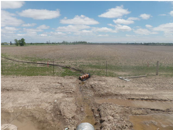
Crossing 12 – Looking downstream
