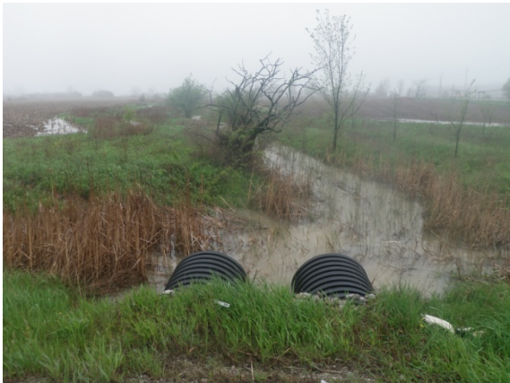
Crossing 6 – Looking upstream
