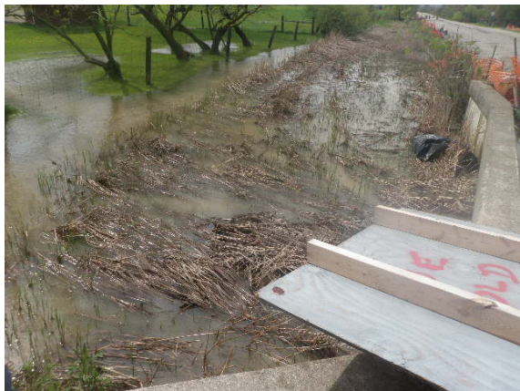
Crossing 11 – Looking upstream
