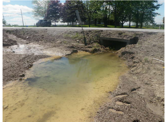
Crossing 14 – Downstream facing culvert
