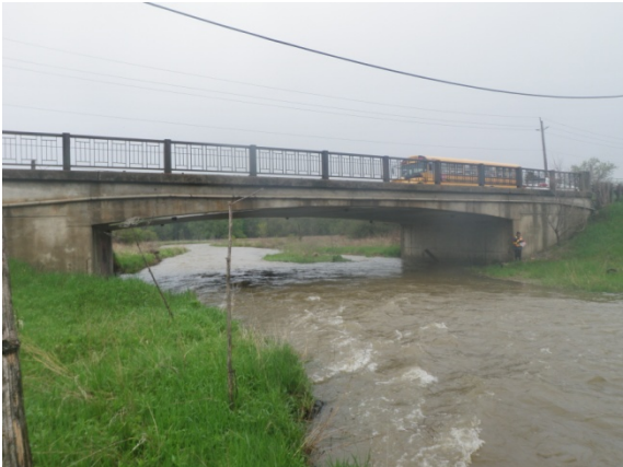
Crossing 7 – Looking downstream
