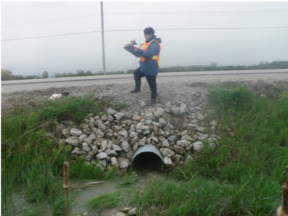
Crossing 8 – Upstream facing culvert
