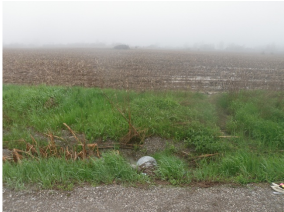
Crossing 5a – Looking upstream
