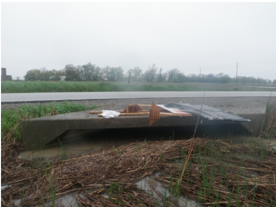
Crossing 3 – Downstream facing culvert
