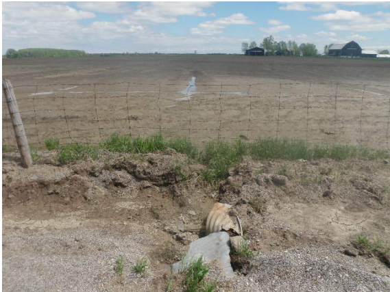
Crossing 13 – Looking downstream
