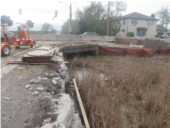
Crossing 11 – Downstream facing culvert
