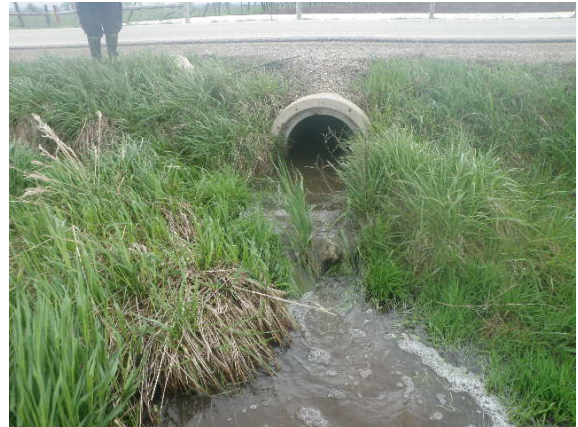
Crossing 10 – Downstream facing culvert
