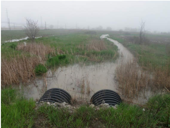
Crossing 5a – Looking downstream
