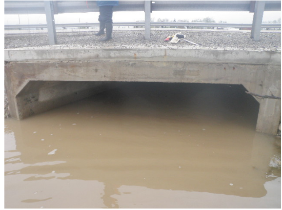
Crossing 9 – Looking downstream
