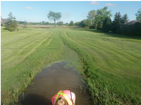
Crossing 16 – Looking downstream
