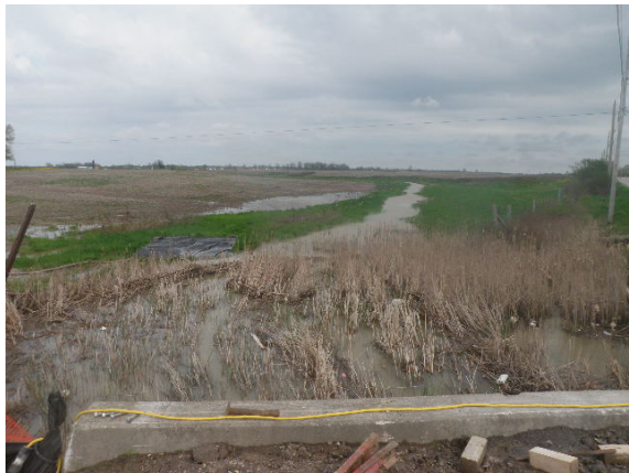
Crossing 11 – Looking downstream
