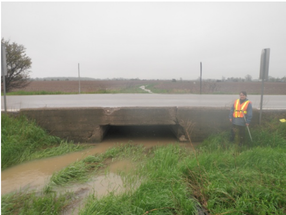
Crossing 1 – Upstream facing culvert
