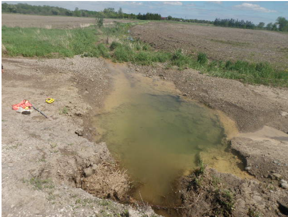
Crossing 14 – Looking downstream
