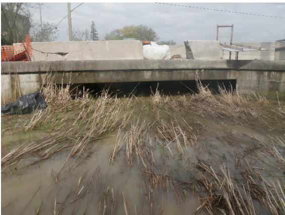
Crossing 11 – Upstream facing culvert
