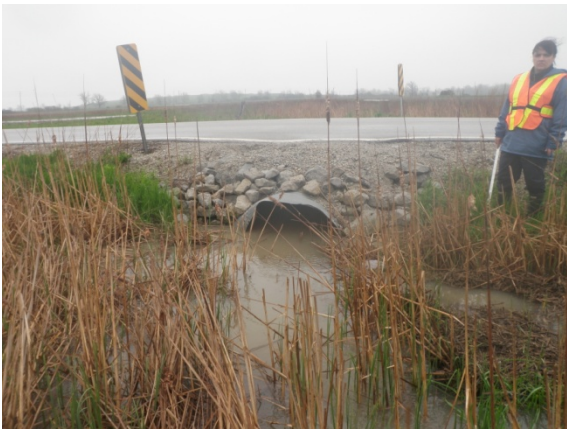
Crossing 2 – Upstream facing culvert
