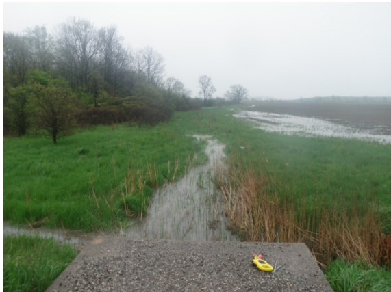
Crossing 5 – Looking downstream
