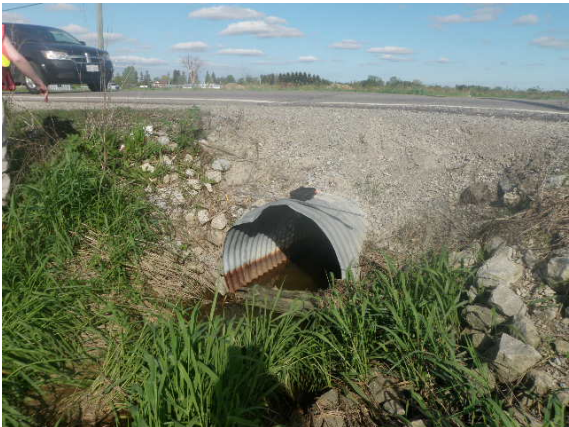
Crossing 17 – Upstream facing culvert
