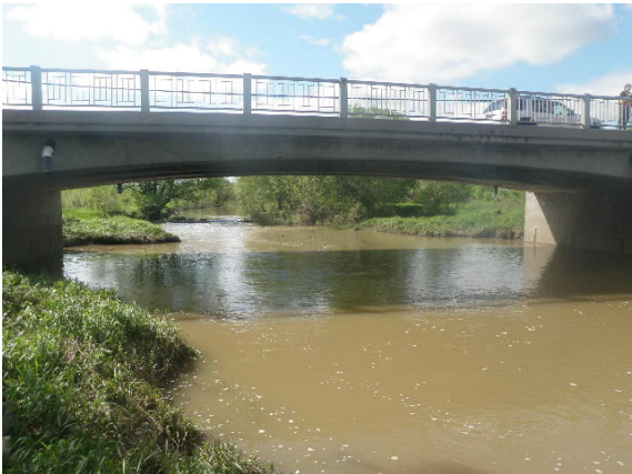
Crossing 15 – Downstream facing bridge
