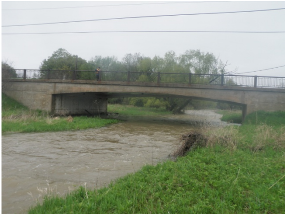
Crossing 7 – Looking upstream
