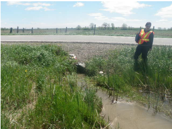
Crossing 4 – Upstream facing culvert
