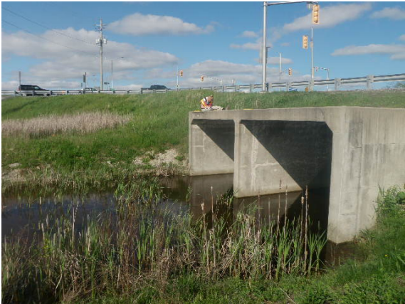
Crossing 18 – Upstream facing culvert
