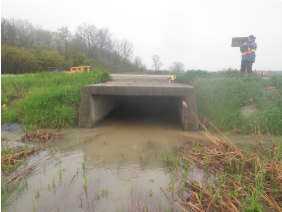
Crossing 5 – Upstream facing culvert
