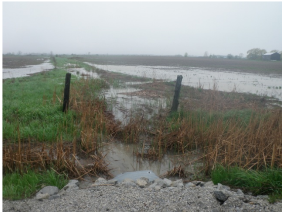
Crossing 2 – Looking upstream
