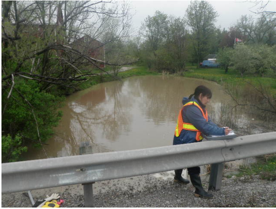
Crossing 9 – Looking downstream
