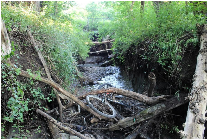
Figure 4-5: Upstream view of severe degradation, scour along the banks, and large woody debris jam
