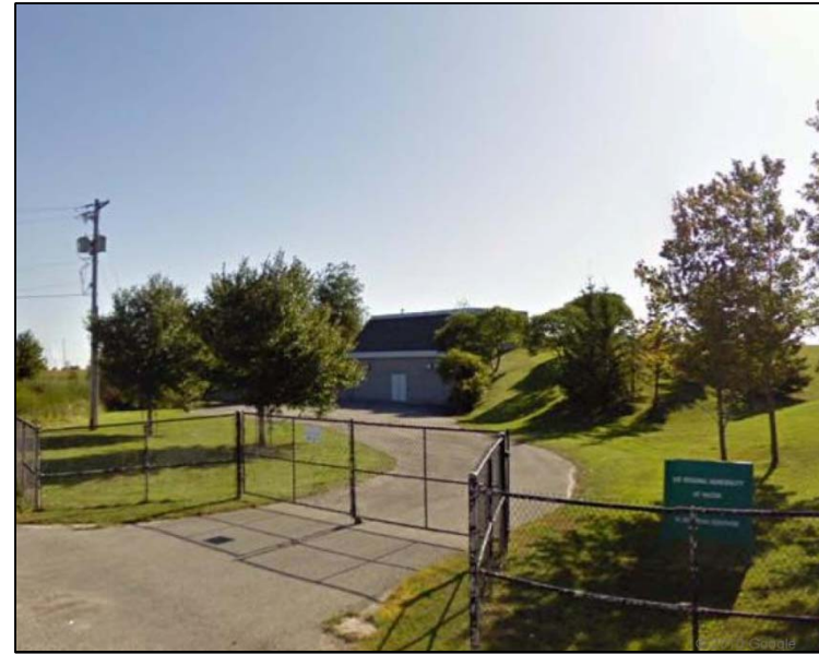
Profile (Street) View – off No. 22 Sideroad
