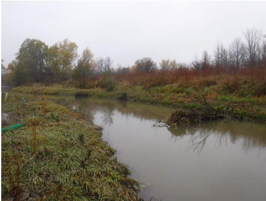
11. View of installed woody debris within restored area of upstream reach (facing north) to provide habitat opportunities for fish within the reach.
