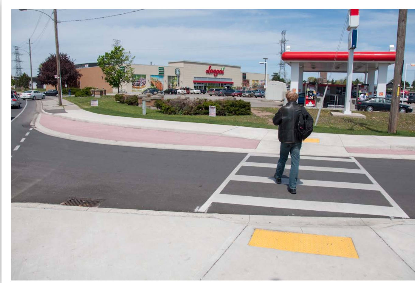
Curb ramps and high visibility crosswalk
