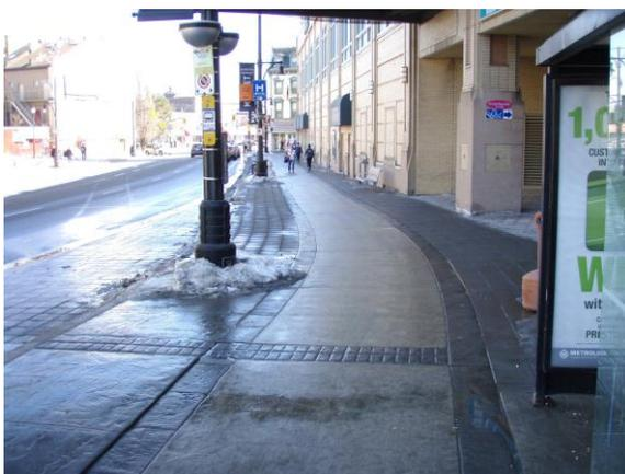
A bus stop detectable strip extends through the sidewalk from shore line to the curb at the bus stop.
