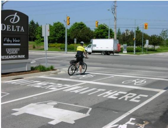
Advanced stop bike box: to allow cyclists to turn left on two-lane, signalized approach, Waterloo ON
