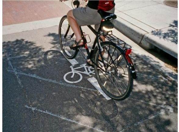
Bicycle lay-by at signalized T-intersection with push-button within reach, Vancouver BC
